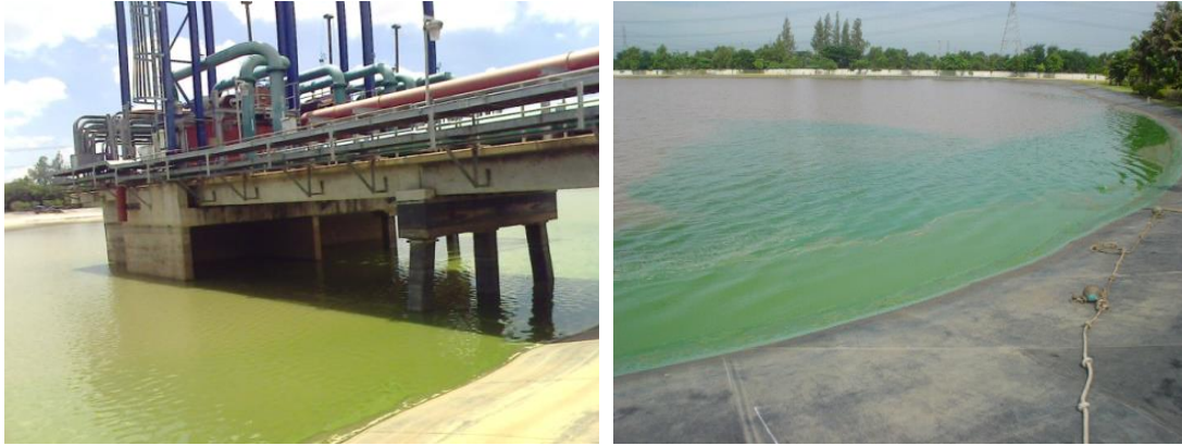
Figure 1.1: Algal blooms in the reservoir of Wang of Wang Noi Power Plant in Bangkok, Thailand (13 June 2011)
