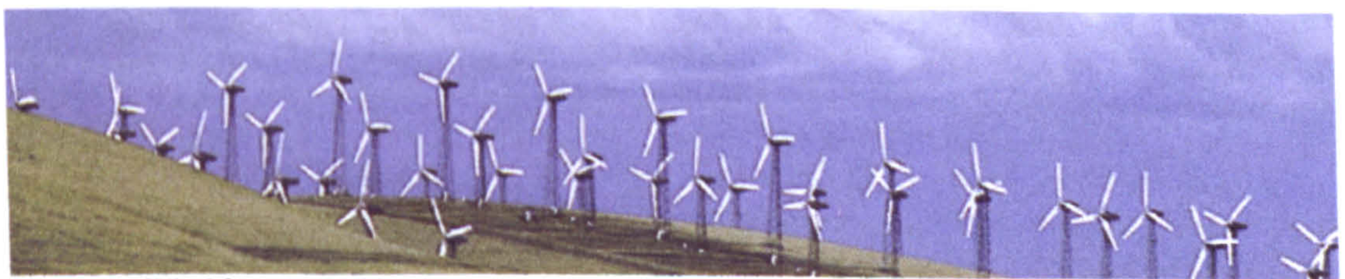
Figure 6.1 Wind farm in California
