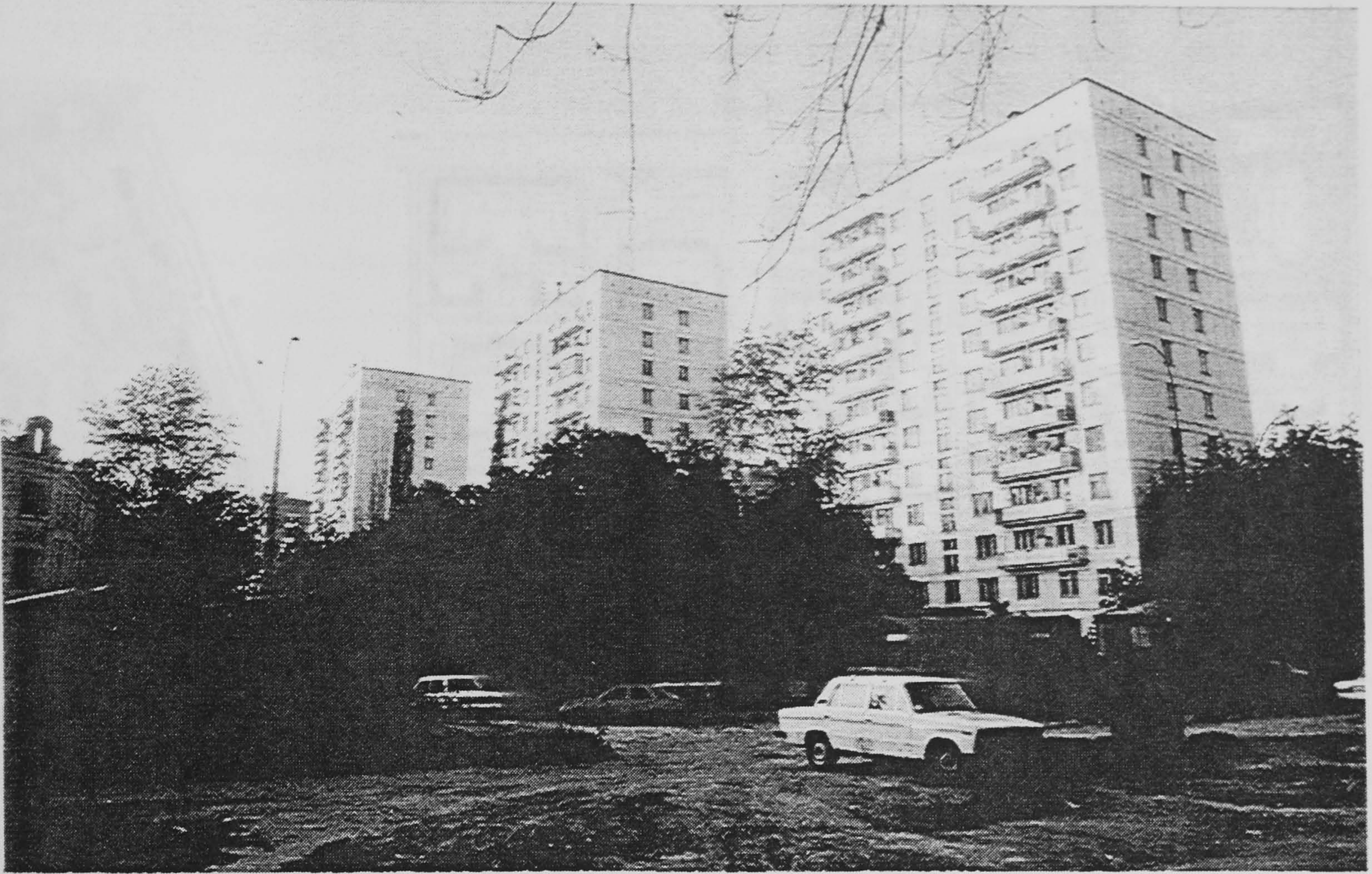
Twelve storey pre-fabricated concrete block housing. Late sixties early seventies
