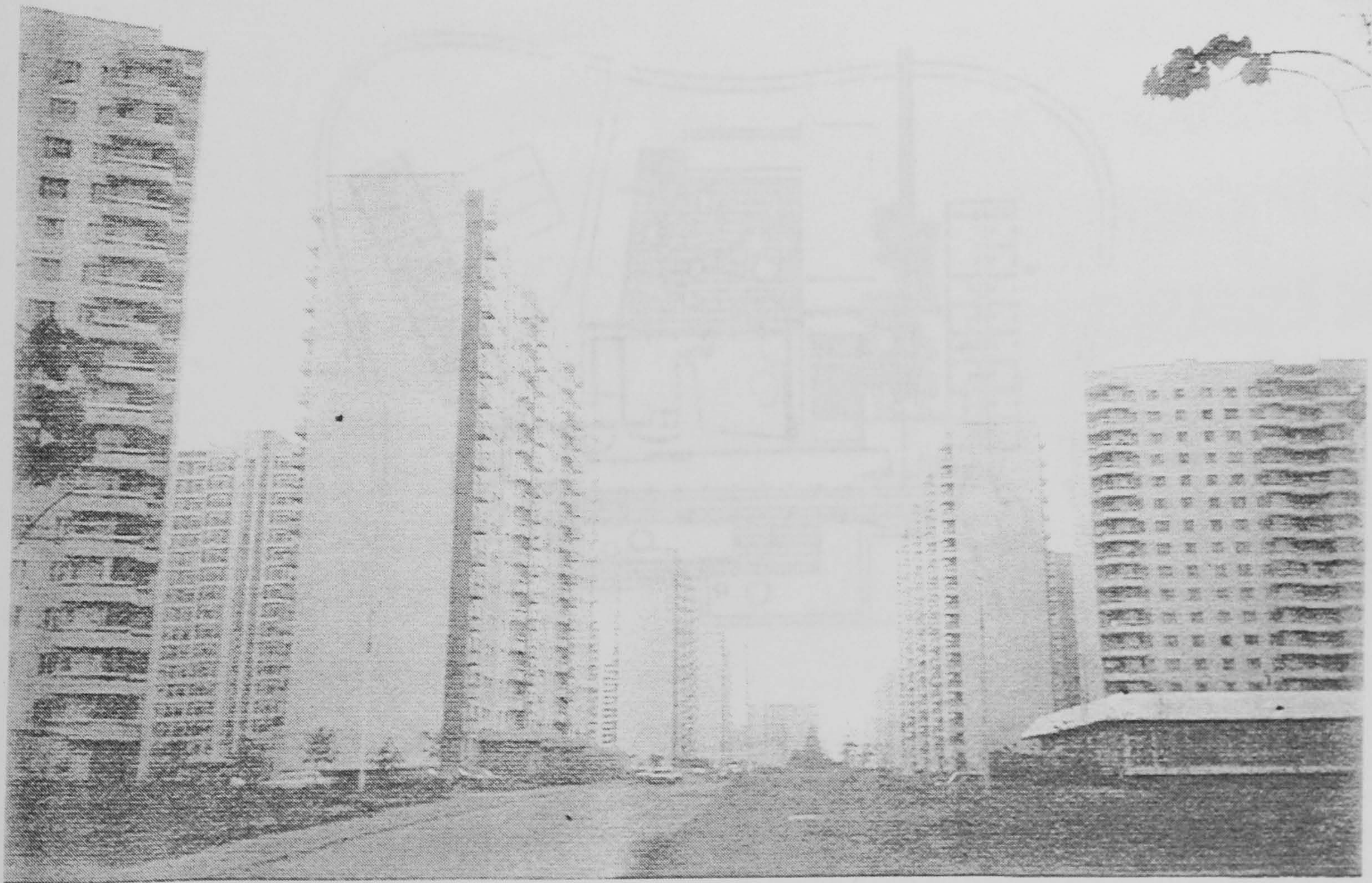
Twenty storey pre-fabricated large concrete panel housing blocks, Moscow
