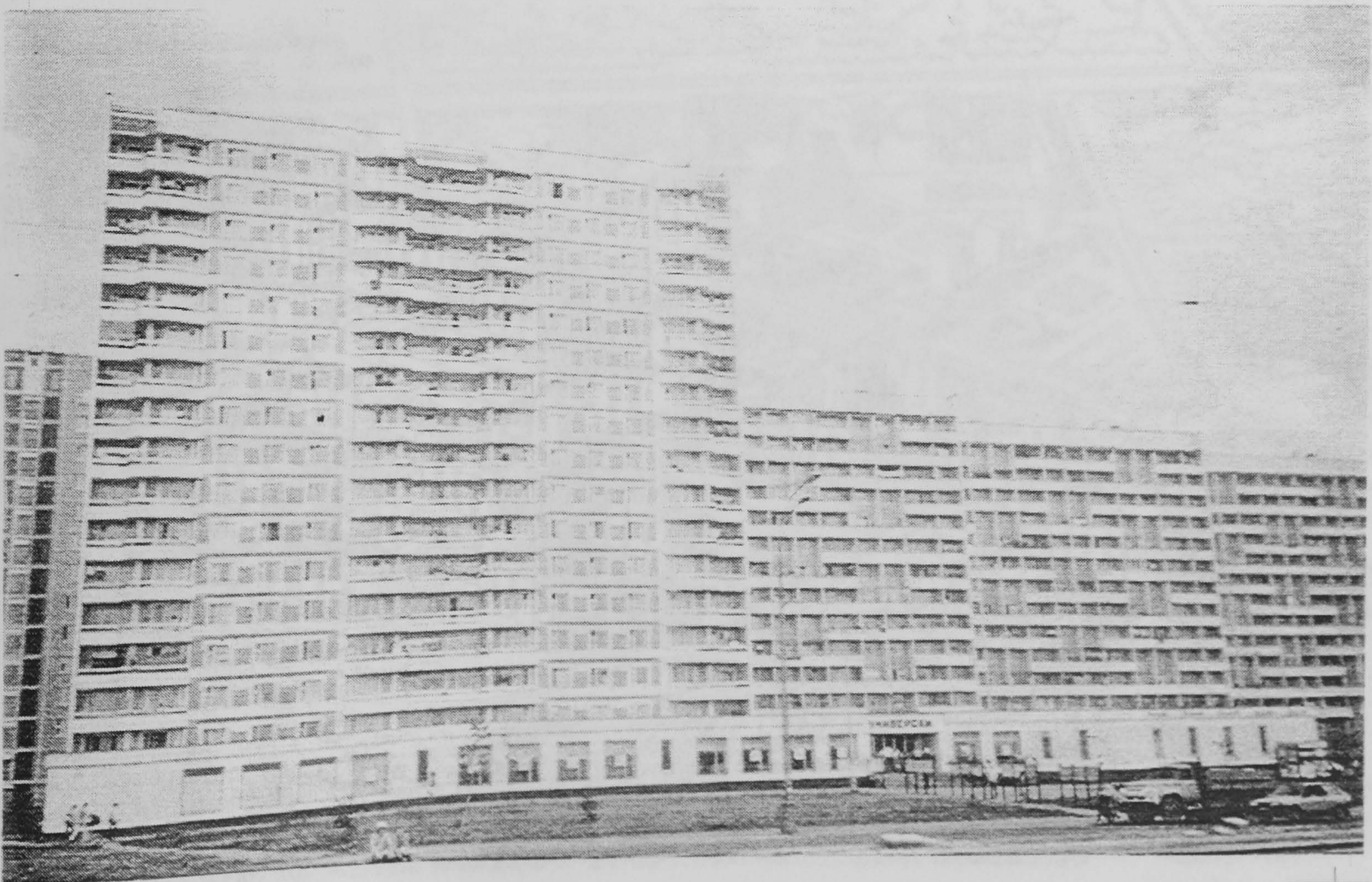
Sixteen storey pre-fabricated concrete panel housing. Late seventies early eighties
