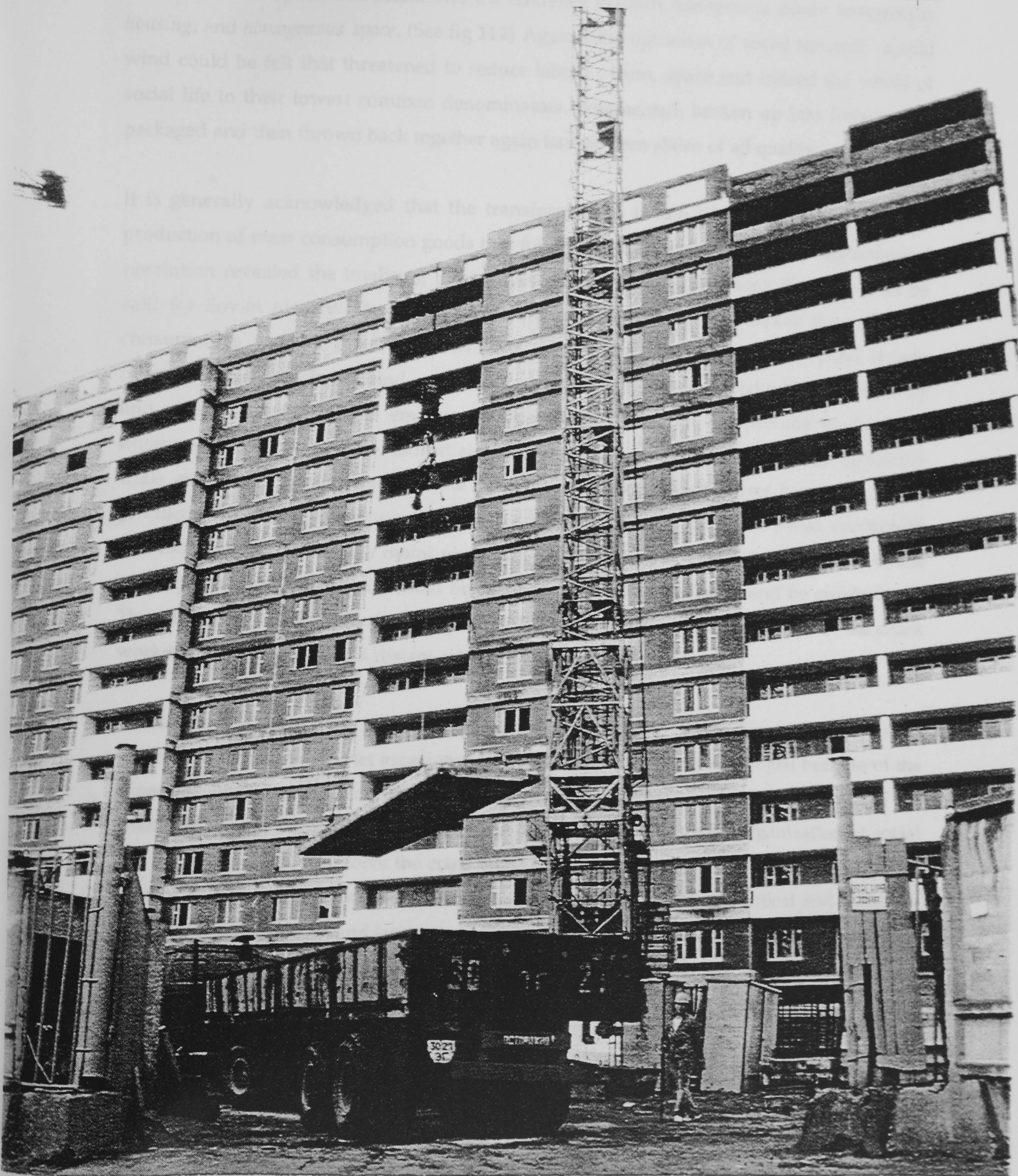
On the building site in 1994
