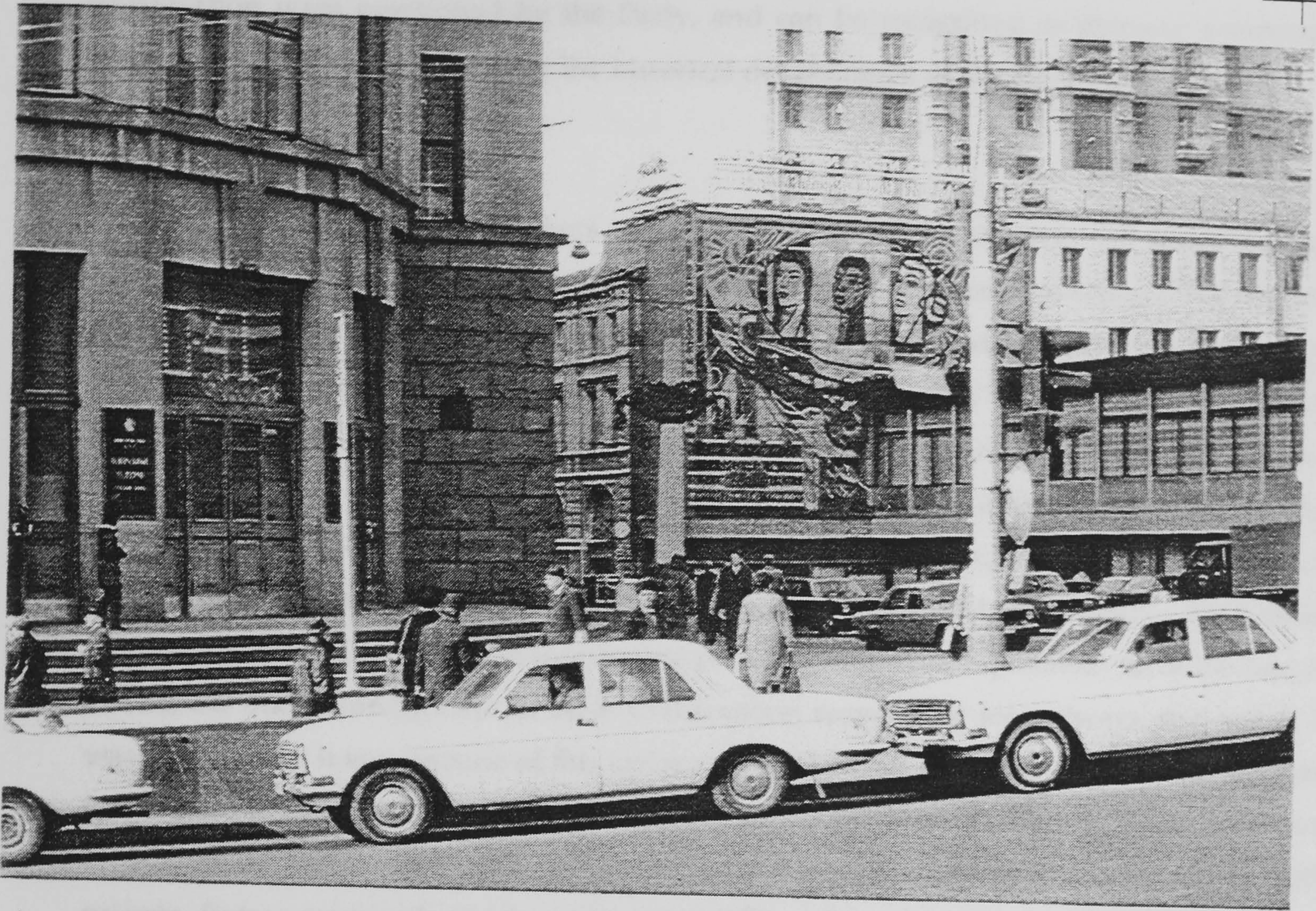
Main entrance to the Central Telegraph Office on Tverskaya Street (In the Soviet era known as Gorky Street)
