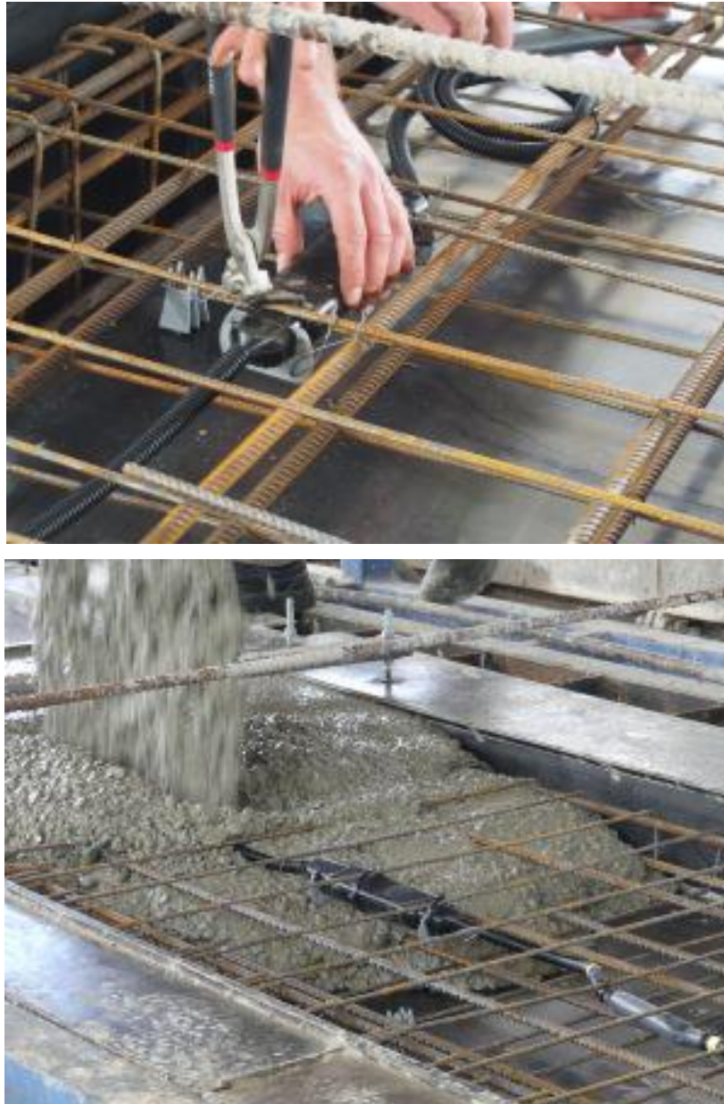
Figure 5-1. Manual deployment of an embedded sensor for a precast grandstand element 168 .
