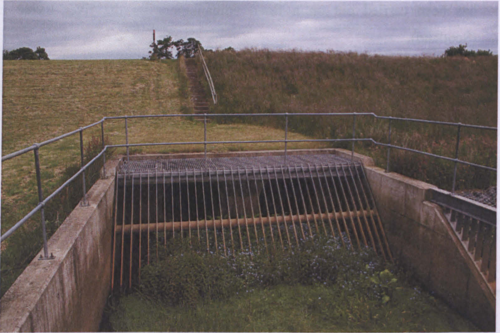
Figure 10.6. State-of-the-art culvert across the flood embankment in Galston.
