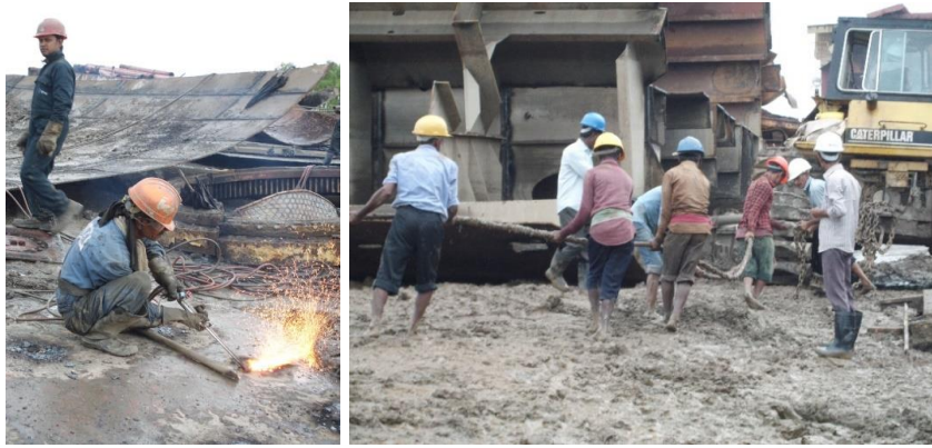
Figure 4.3: Secondary cutting operation and material handling
