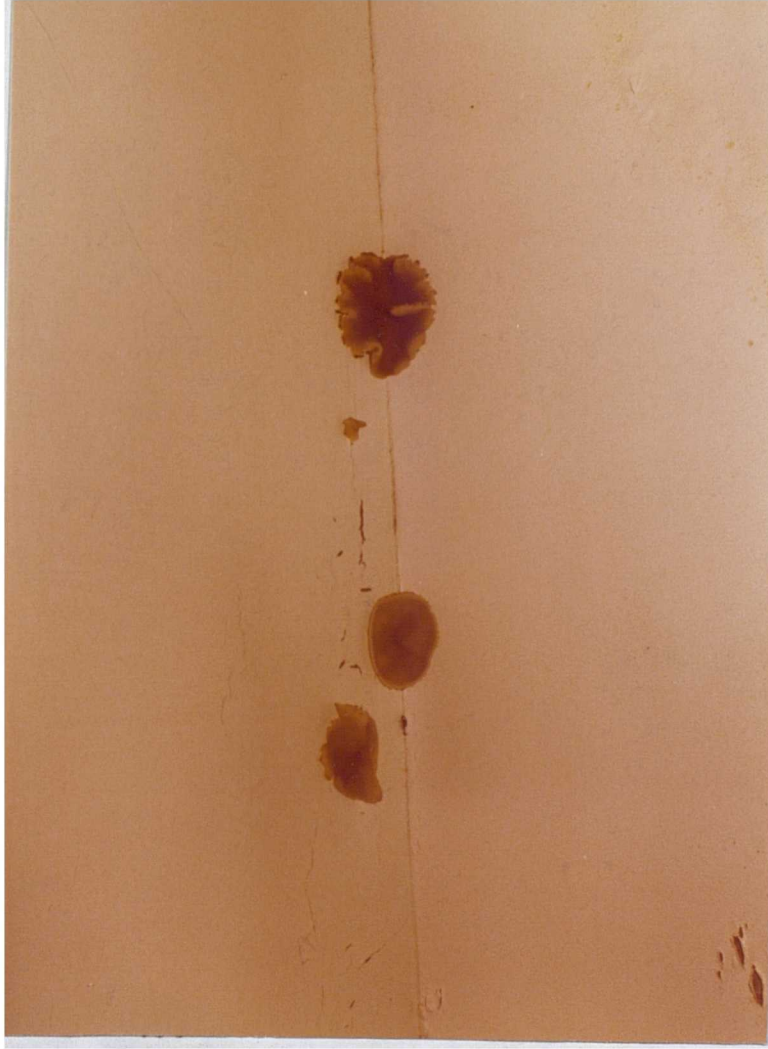
Figure (4.6) Plaster mould damage to the whole plaster layer, showing brown fruit bodies (leathery). Conditions in the bathroom of a centrally heated building, shown above, can be summarized as - unsatisfactory ventilation, high water vapour production with continuous saturation, surface temperature below dew point, and organic materials in the plaster.
