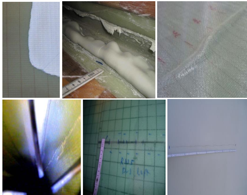
Figure 3.9: Some defects arising from uncontrolled manufacturing processes: void arising from poor infusion (top left); excess bonding resin (top middle); fibre-wrinkling (top right); crack in shear web (bottom left); fibre discontinuity (bottom middle); cracking arising from discontinuity (bottom right), [45]
