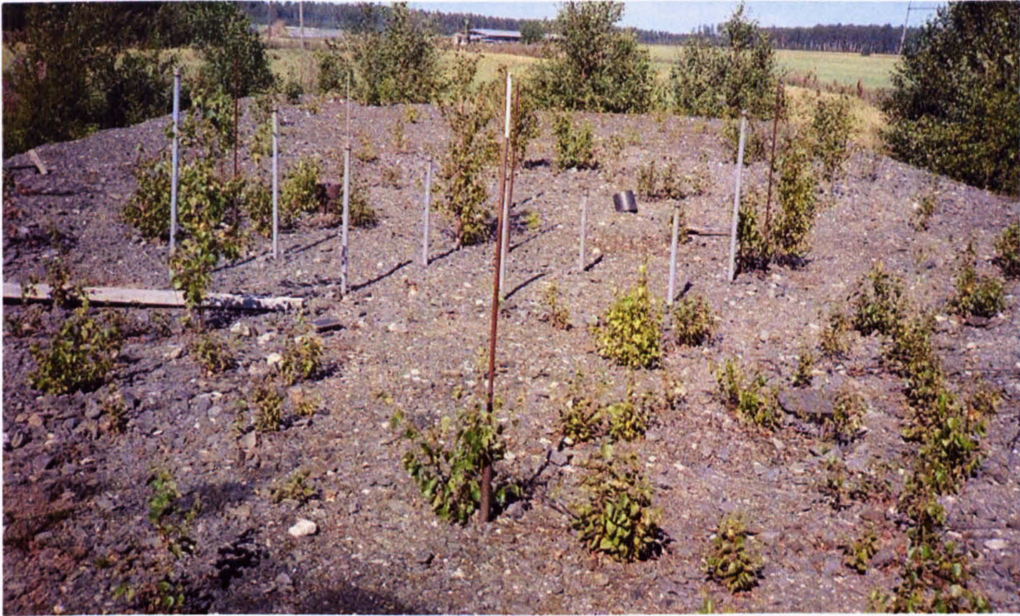
Figure 6.1: Murro test embankment
