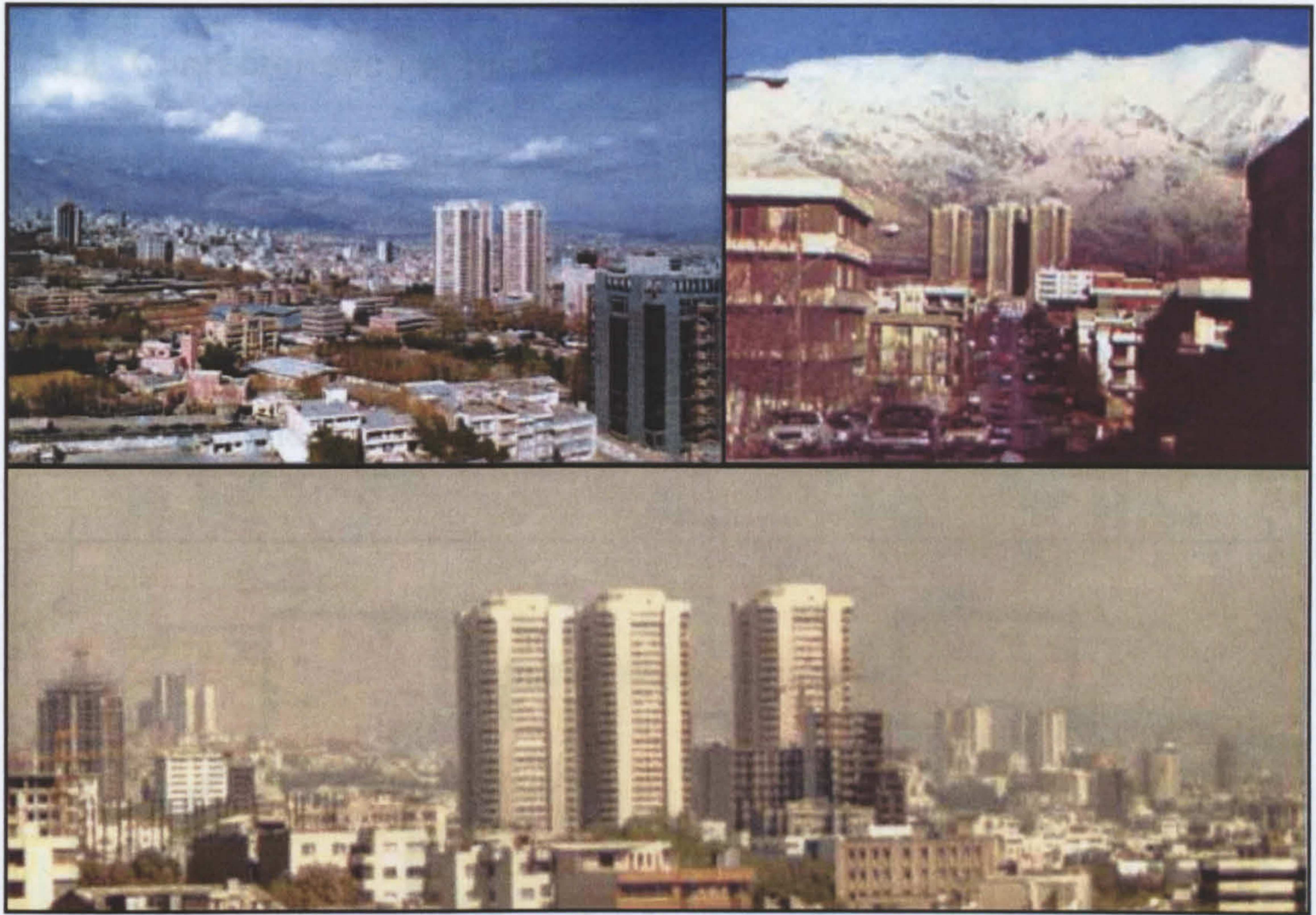
Figure C. 34 Different views of the Eskan inner city residential towers. Source: Author, summer 1994.
