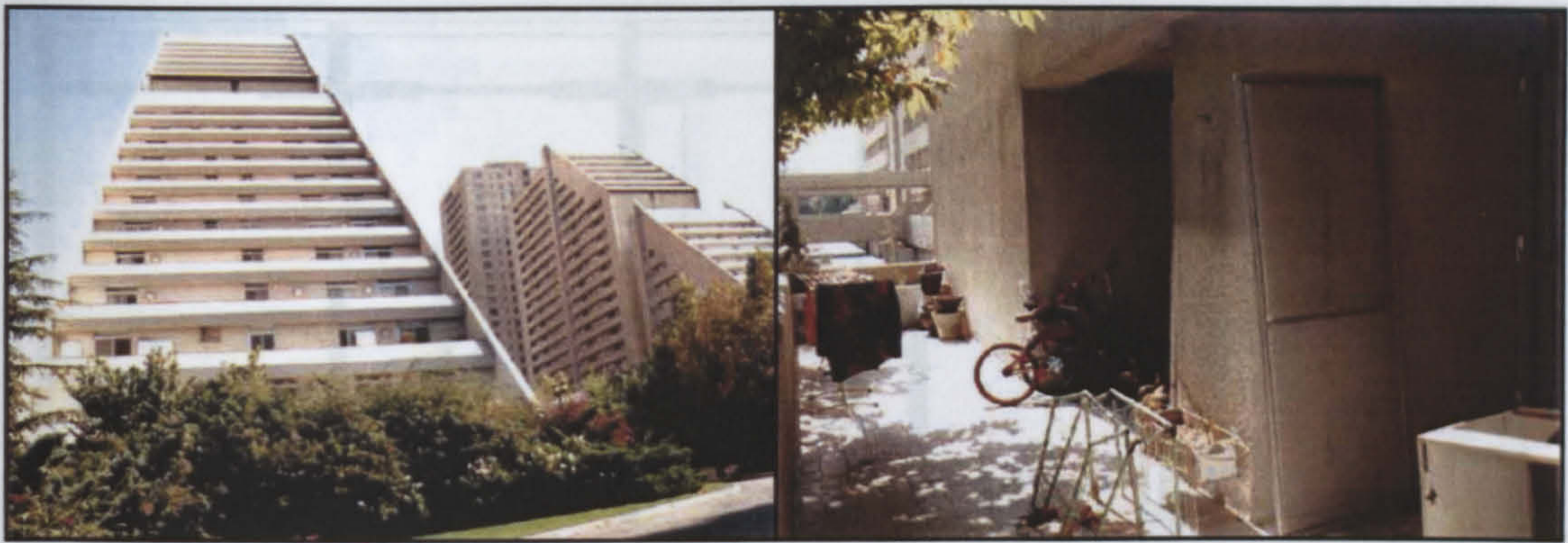
Figure C.28 Internal and external views of balconies.
