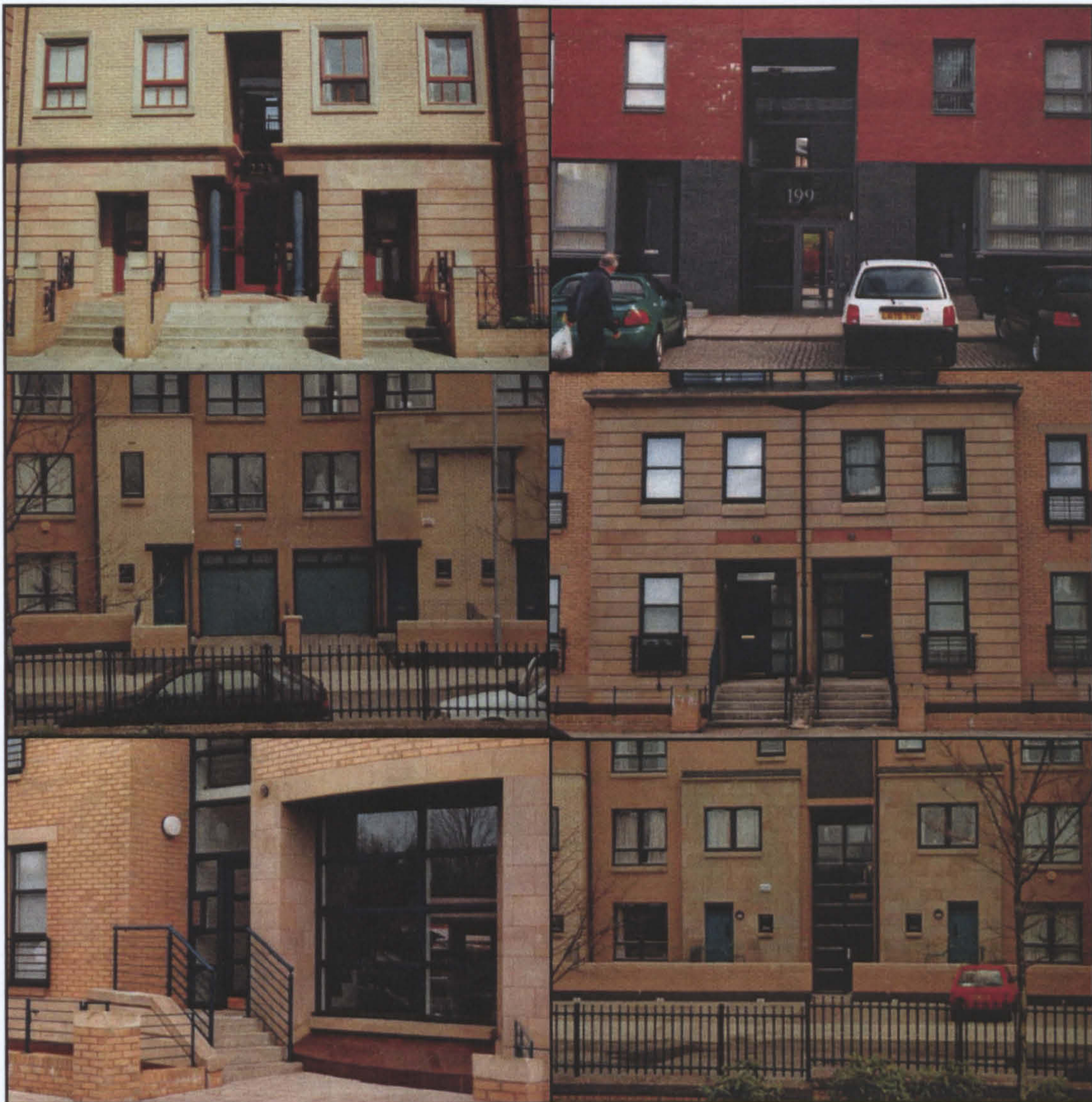
Figure 2. 24 Variety of entries designs to the buildings.
