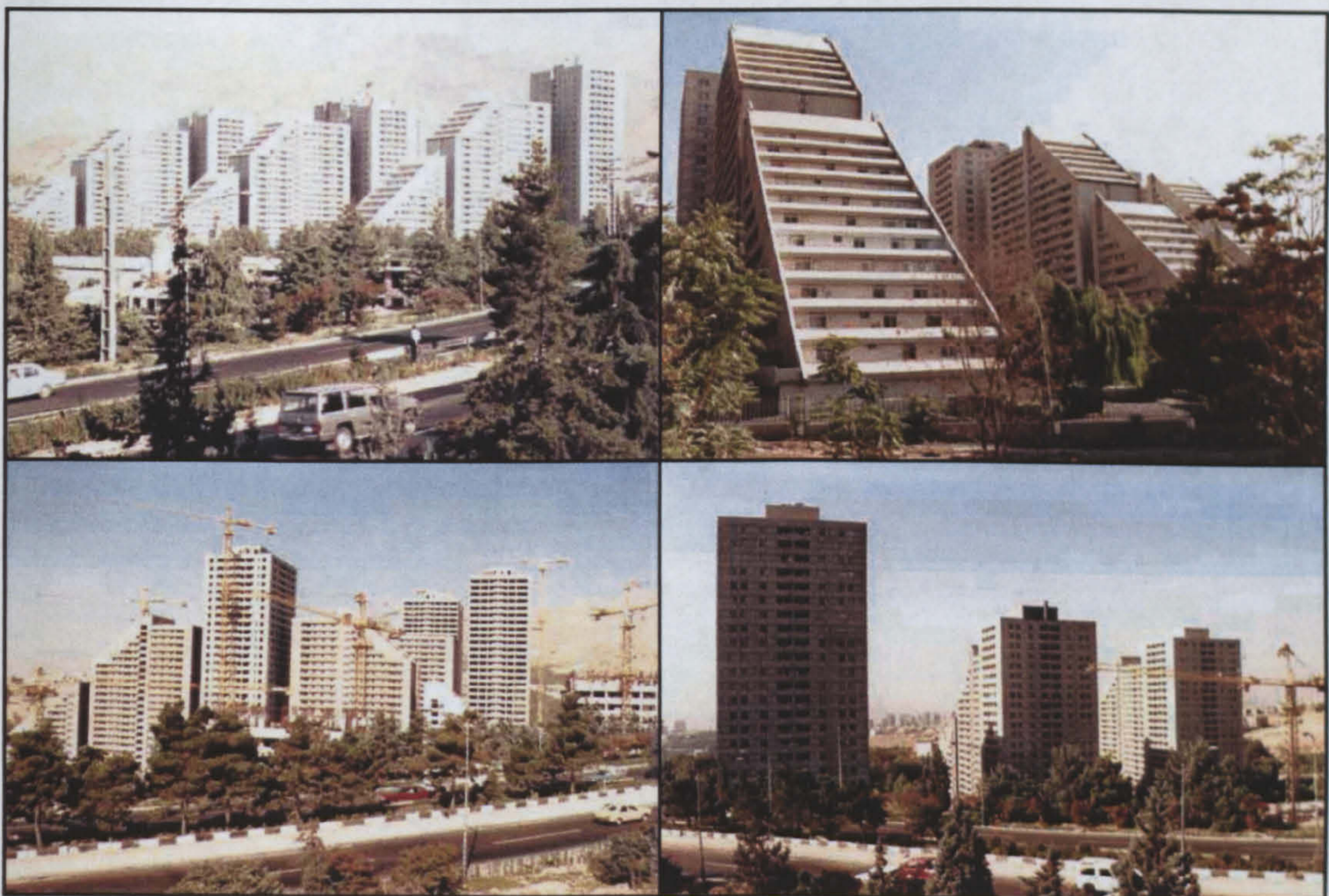
Figure C. 19 Different angles views of the Atisaz residential buildings.
