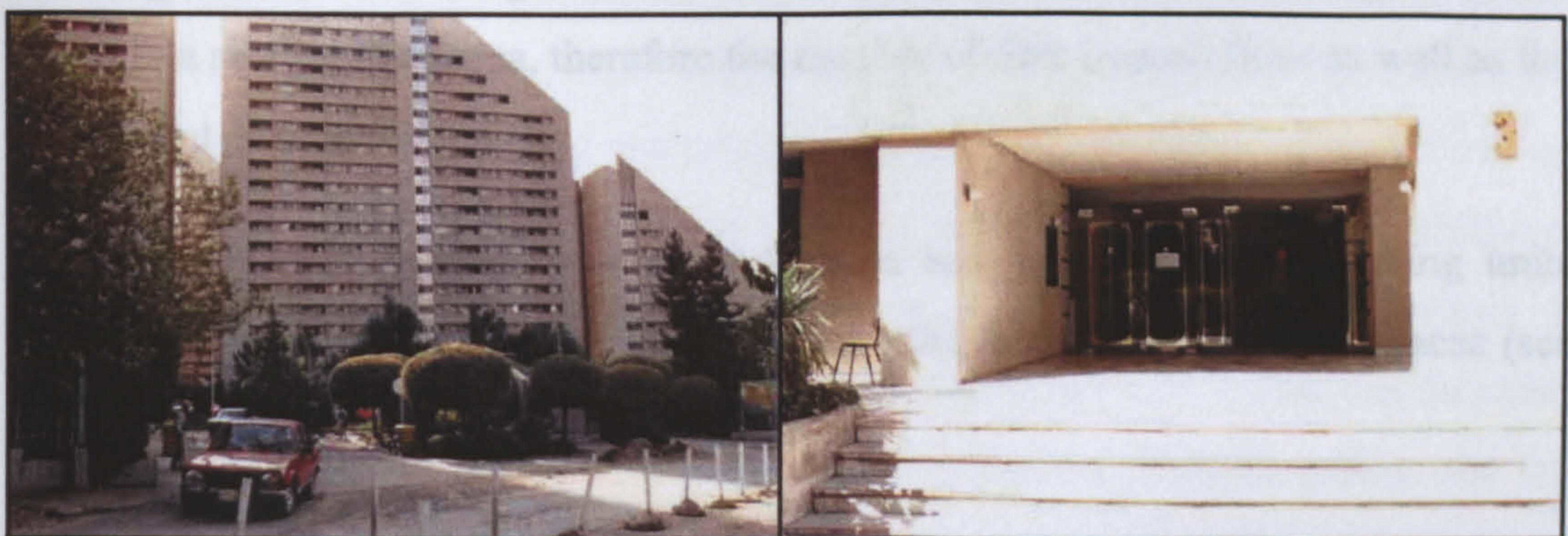
Figure C. 26 Access to the housing is closely monitored/controlled by bars at entry gate of the scheme as well as a lobby-man in each building.
