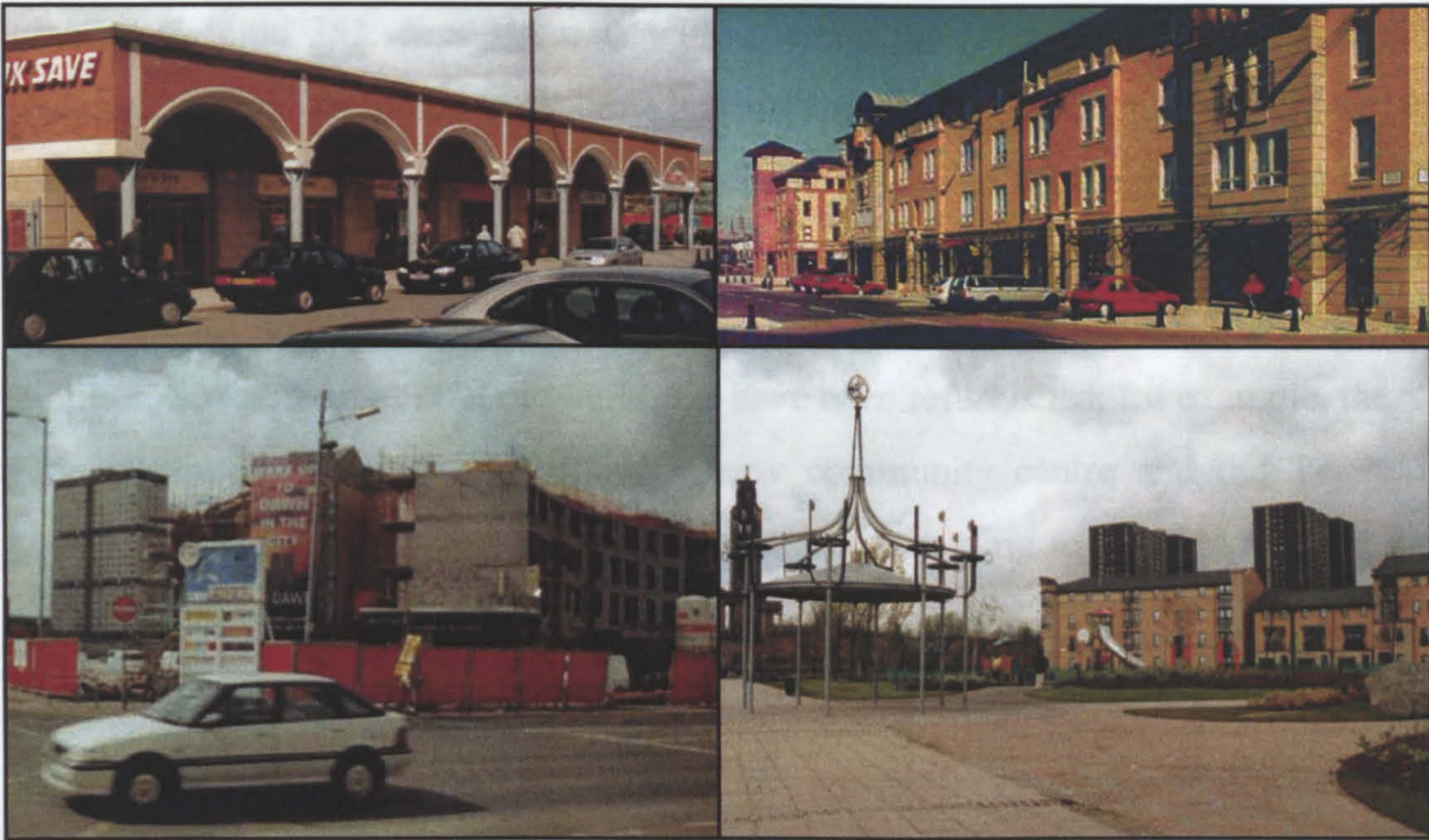
Figure 2. 21 (Top/L) Shopping Centre, (Top/R) Individual shops -ground floor, (Bottom/L) Hotel - under construction, (Bottom/R) Gorbals Park. Source: The author, April 2000.
