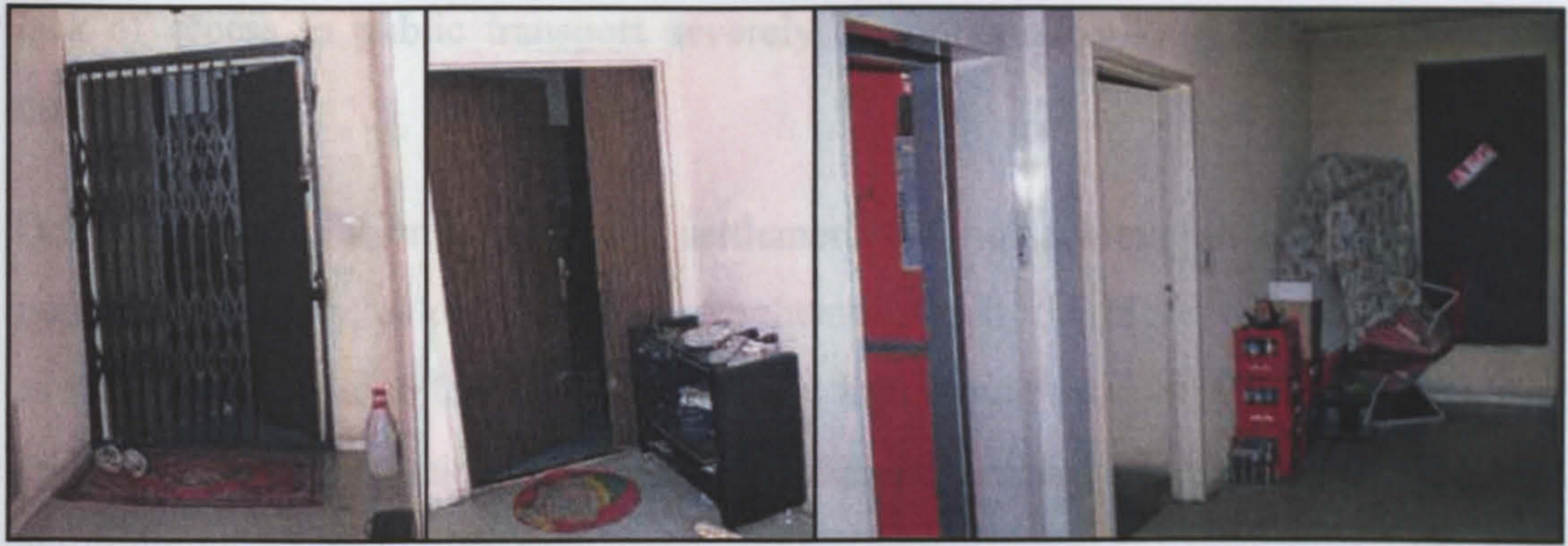
Figure C. 16 Typical view of the corridor and entry doors to dwellings.
