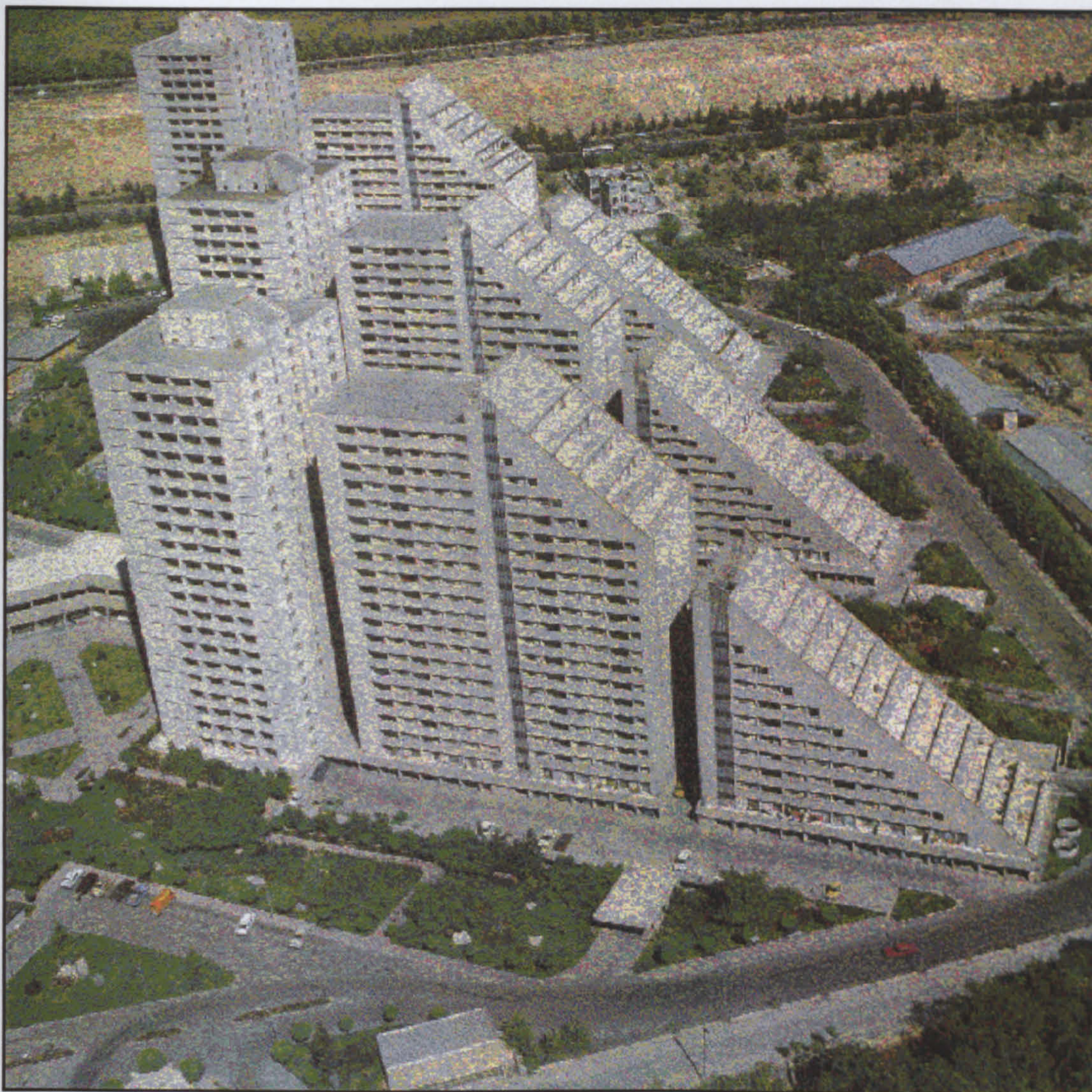
Figure C. 20 A western view of phase one buildings illustrating the Chamran expressway to east of the scheme (behind the buildings), main entry point to the scheme to the west of the scheme, ring roads around the buildings, and on-site and under building parking.
