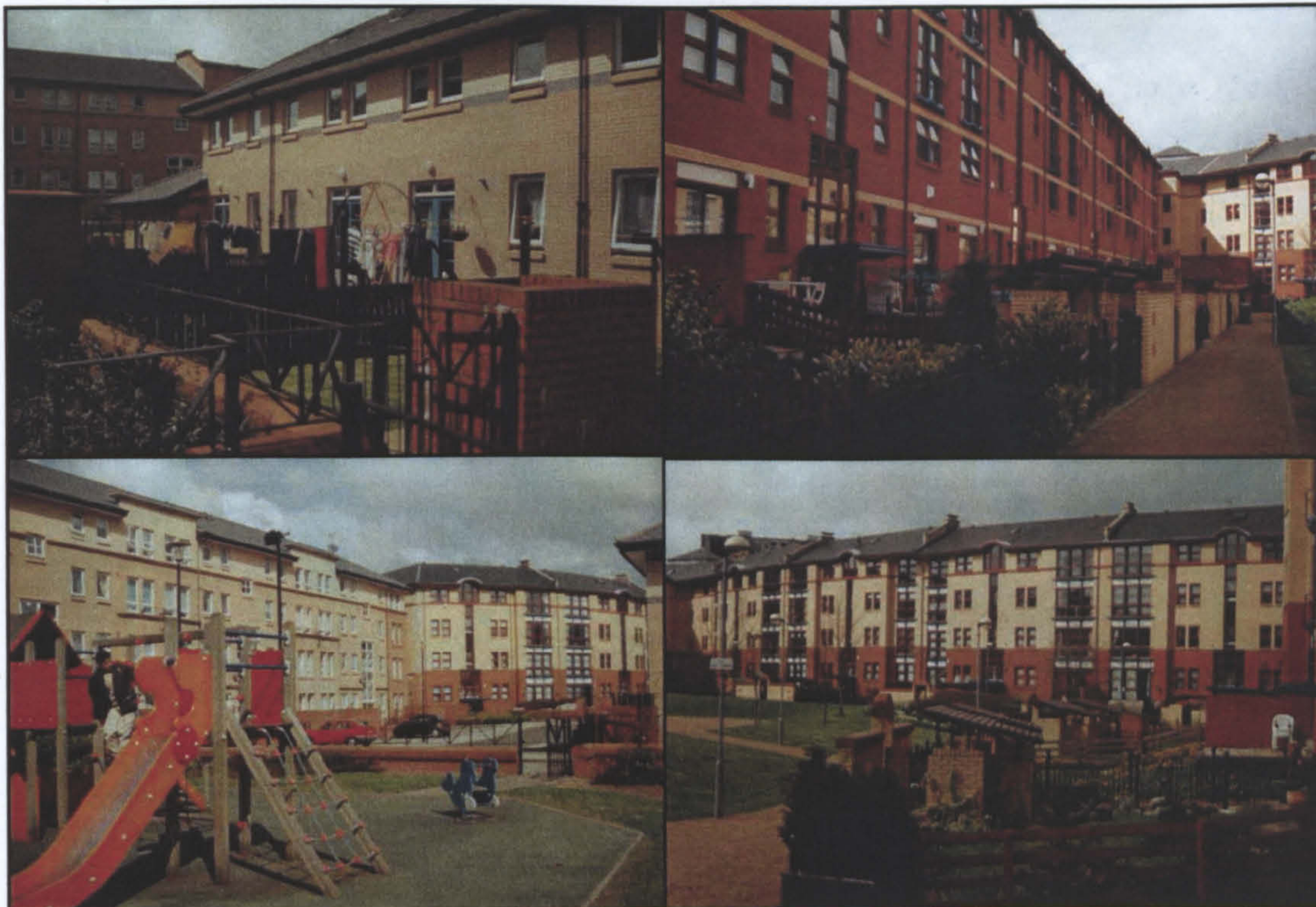
Figure 2.16 The landscaped shared communal space within the block. Source: the Author - April 2000.
