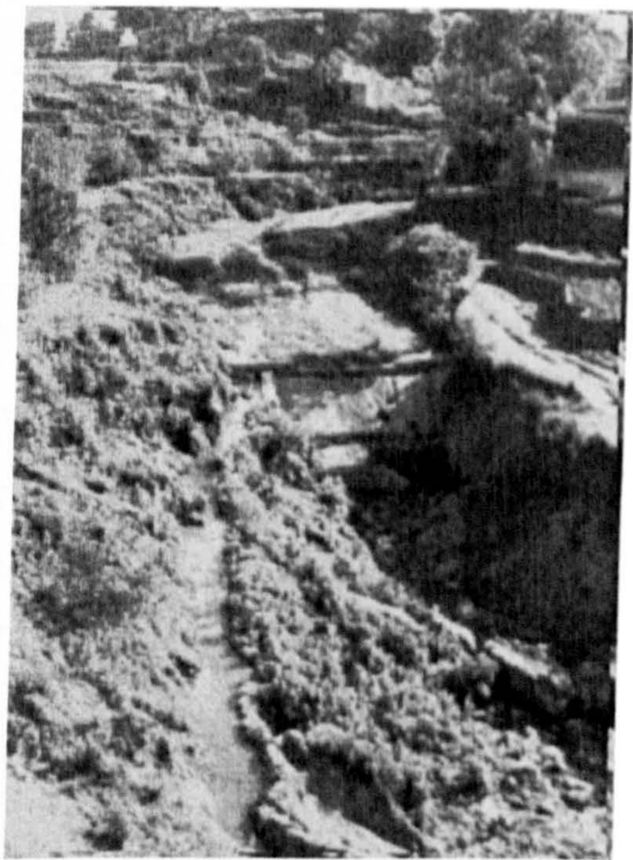
Stream Diverted for Intake
