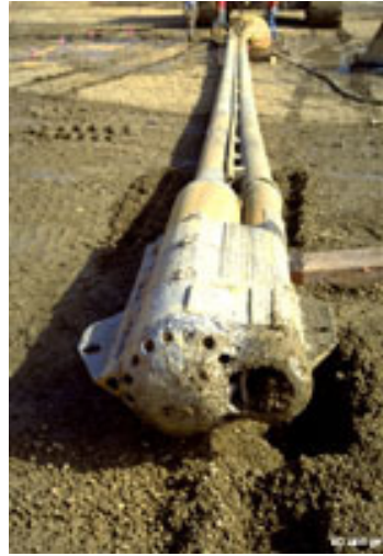
Figure 3.1: End of vibrator with two tubes (Boulangier & Duncan, n.d.).
