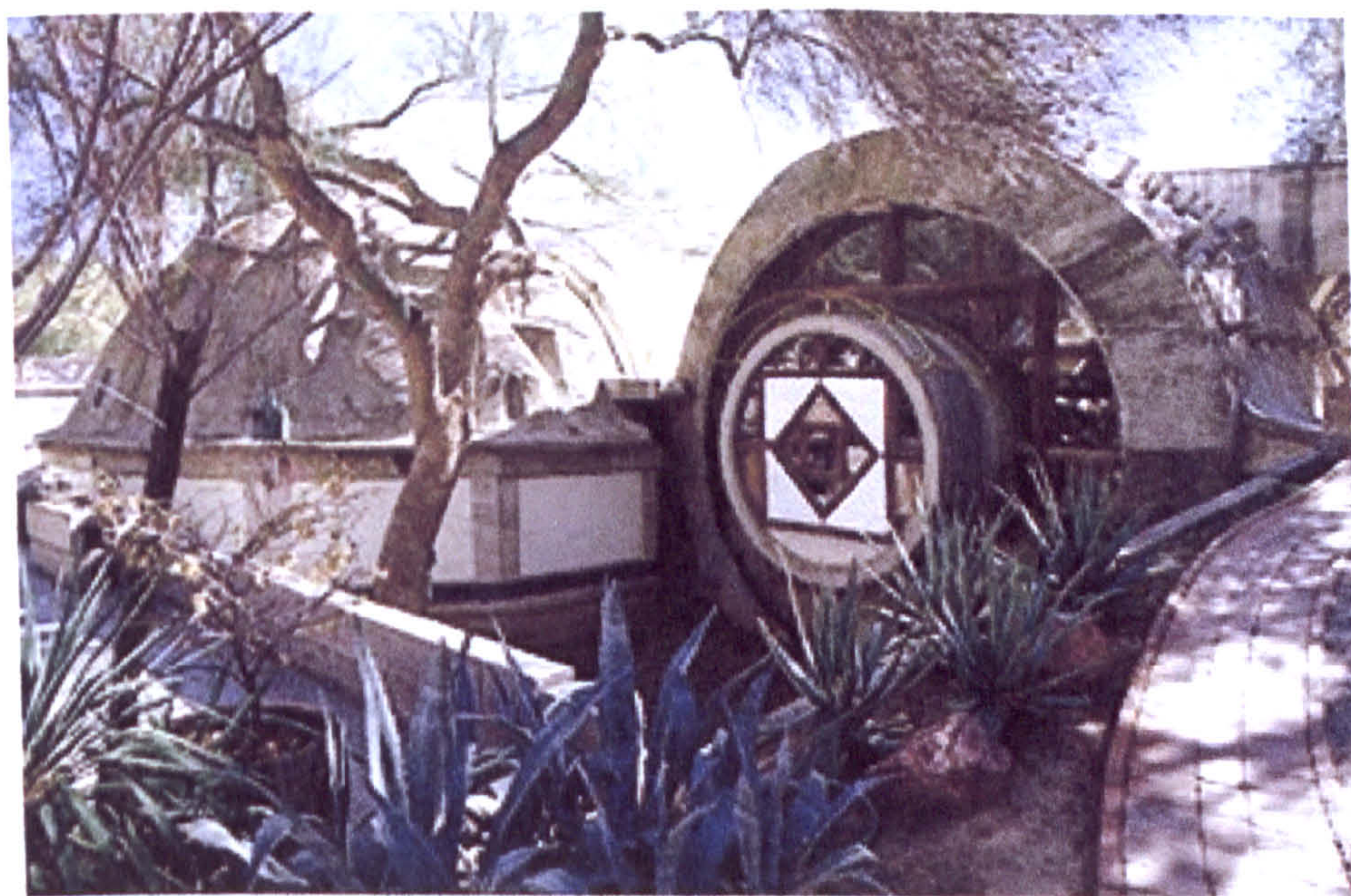
Plate 23 The Pumpkin Apse and Barrel Vaults (1967 - 71)
