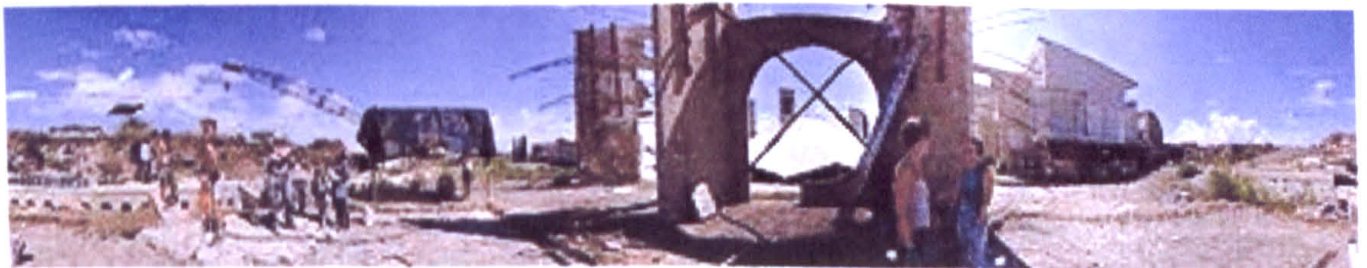
Figure 9.1 Arcosanti: East Crescent under construction, 1999
