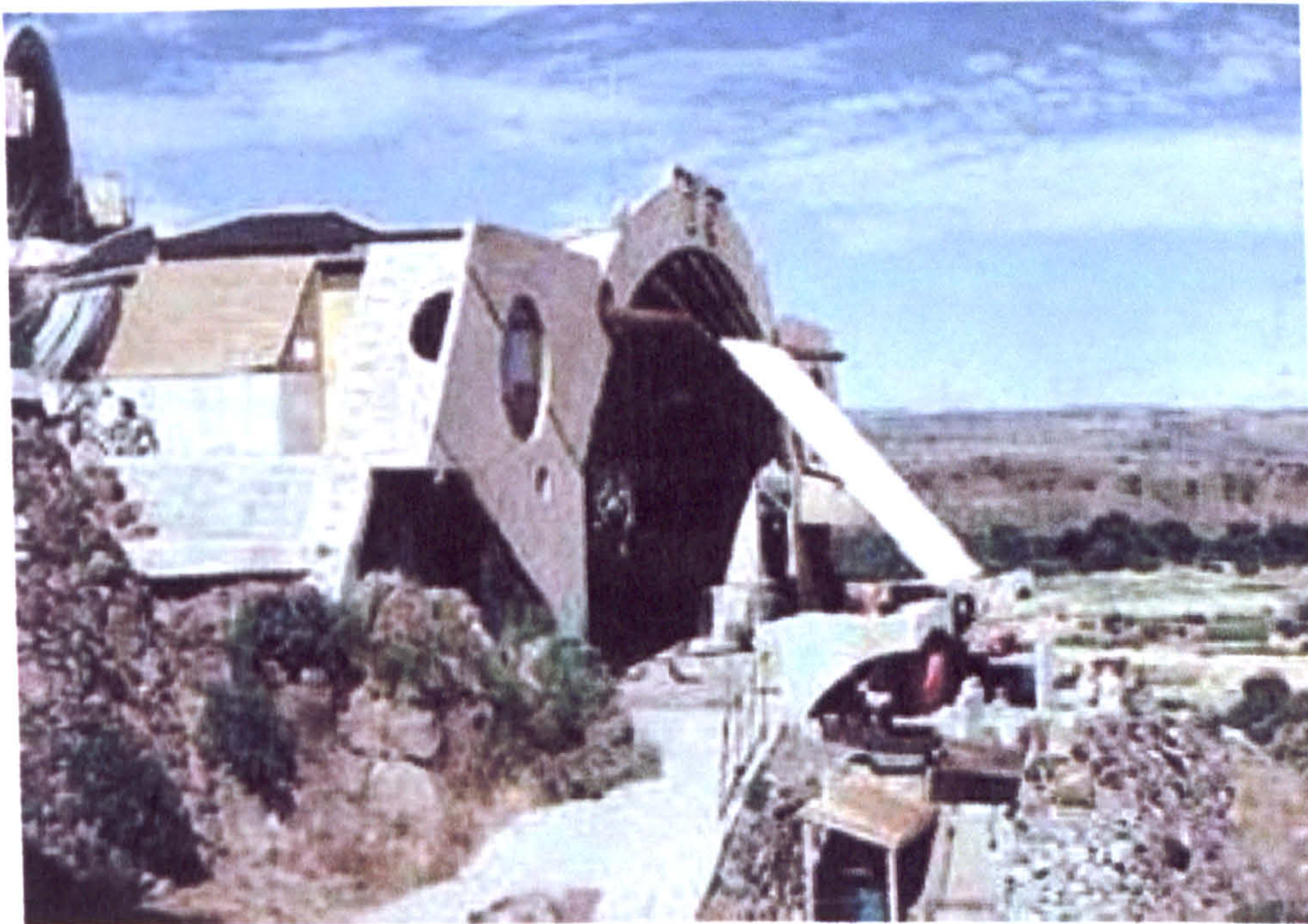
Plate 29 The Foundry Apse (1972 - 74)
