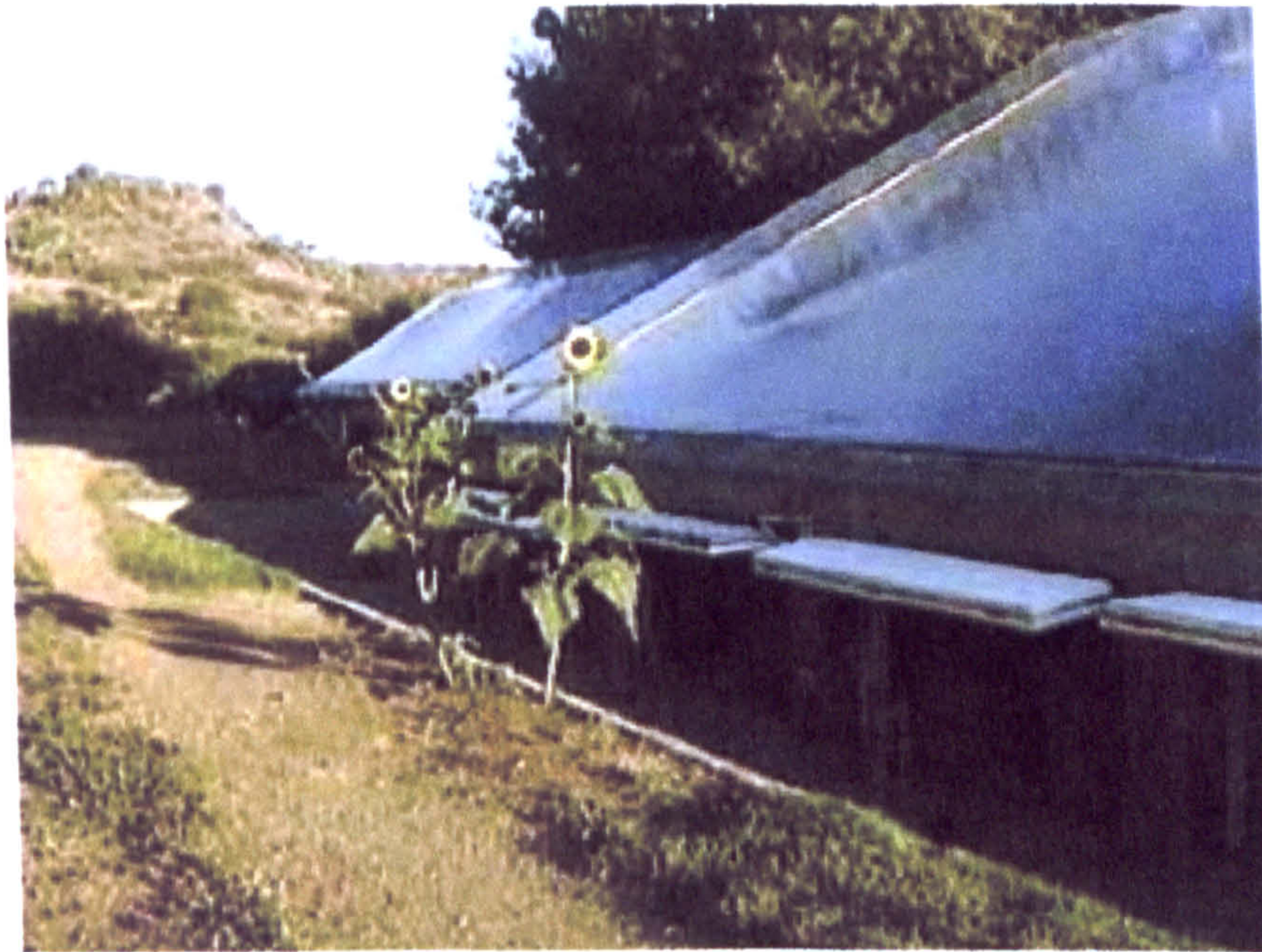
Plate 38 Prototype greenhouses at Arcosanti
