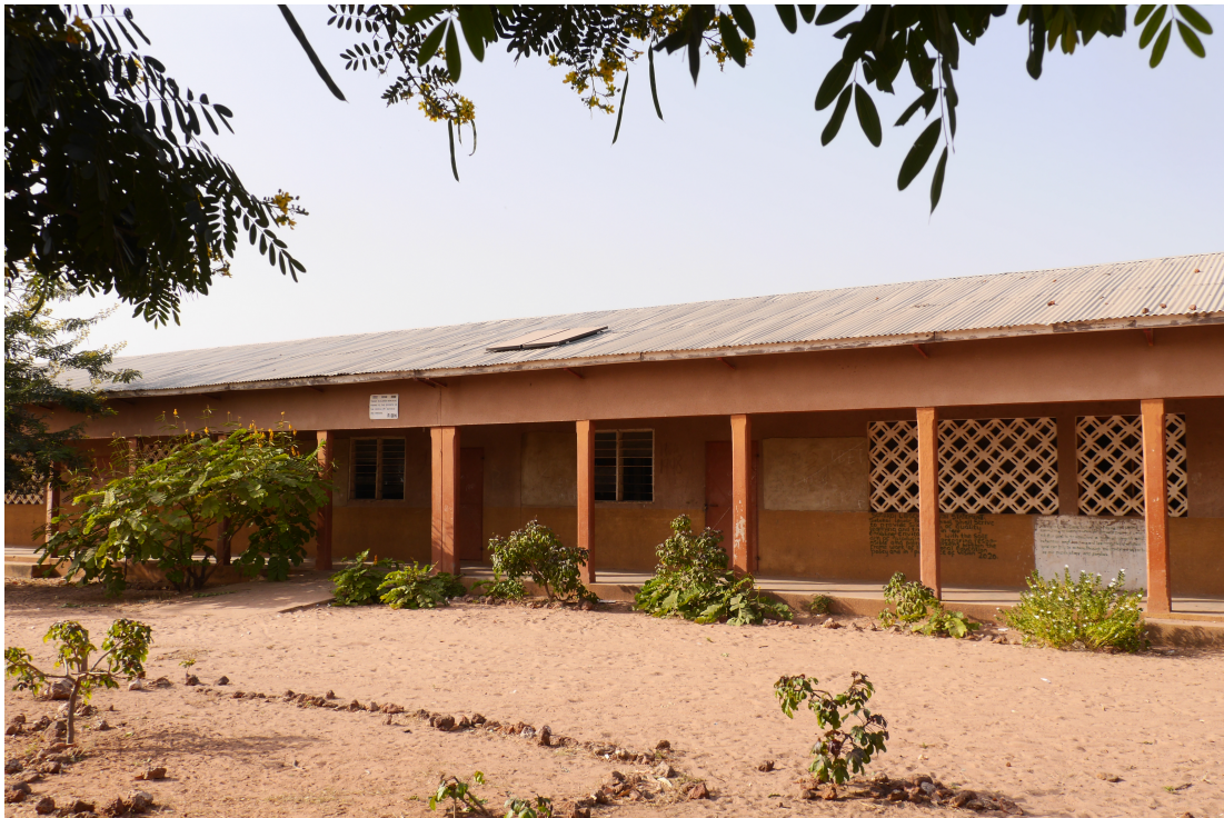
Figure 3.14: Solar PV Project at Sambel Kunda, The Gambia
