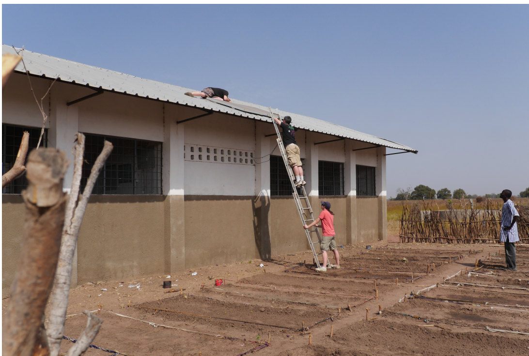
Figure 3.20: Sotokoi Lower Basic Primary under repair
