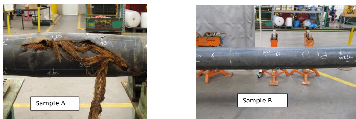
Figure 4-7: Sample description of the investigated flexible pipe
