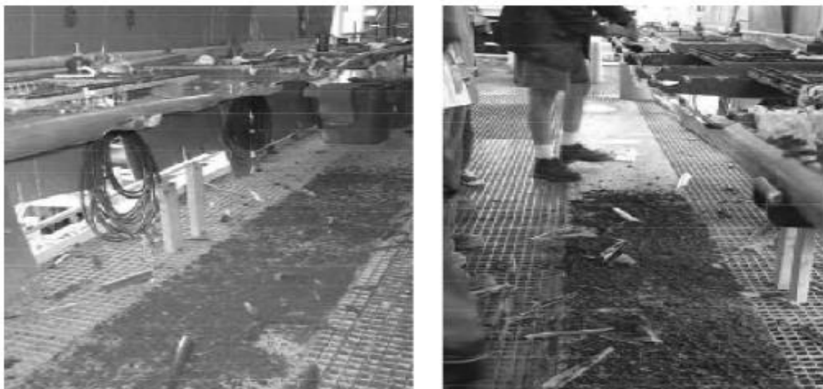
Figure 2-25: (a) Burst pipes on hydrate formation (b) Eliminating clogging in pipes [33]
