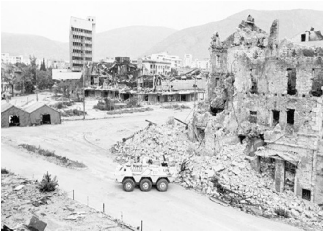
Figure 3-8. Destruction of Mostar (Arna, 2014).
