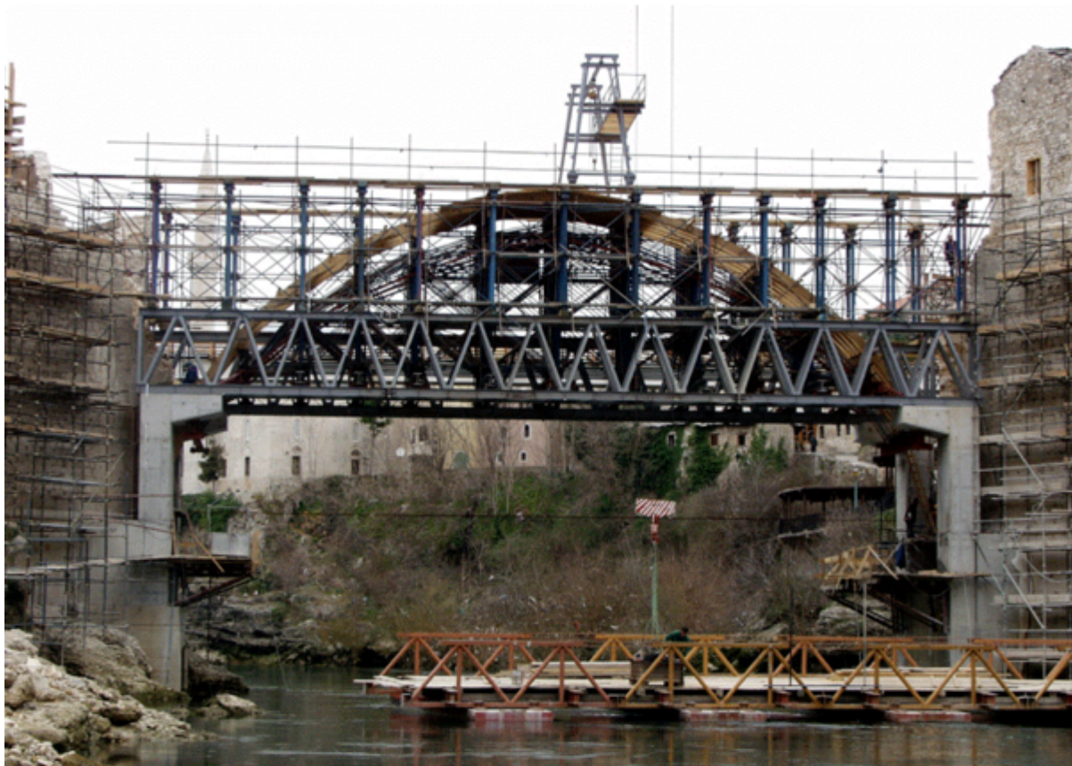
Figure 3-9: Stari Most rebuilding (Colak, 2016).
