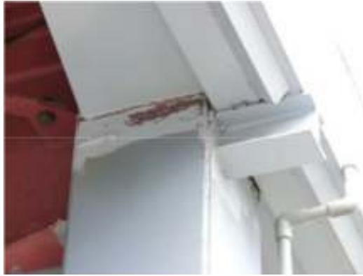
Plate 2.13 Yielding of an older built-up column (Midorikawa et al, 2012)
