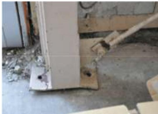
Plate 2.20 Fracture of anchor bolts, out-of-plane deformation of base plate (Midorikawa et al, 2012)
