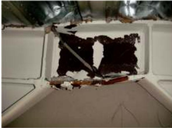
Plate 2.7 Fractured EBF active link in top level of EBF system (Clifton, 2011)
