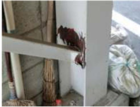
Plate 2.16 Yielding of column web near bracing connection
