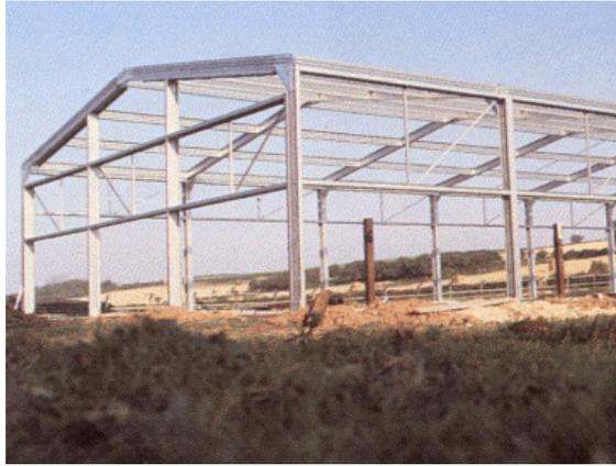
Plate 1.1 General view of a light gauge steel portal frame (IPL, 2011).
