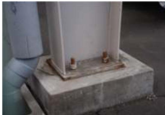
Plate 2.18 Elongation of anchor bolts in an exposed base plate
