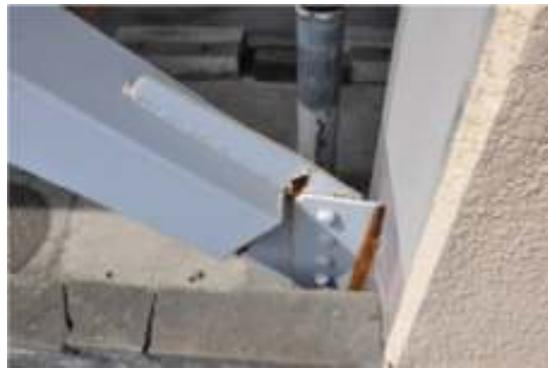
Plate 2.17 Out-of-plane deformation of gusset plate caused by compression
