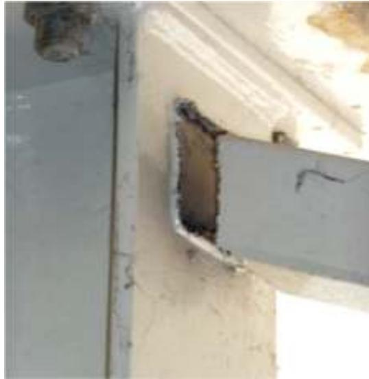
Plate 2.10 Fractured non-ductile brace-to-column connection (Clifton, 2011)
