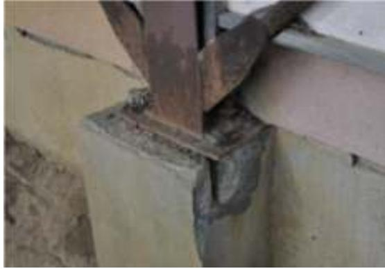
Plate 2.19 Spalling of reinforced concrete foundation supporting a column base (Midorikawa et al, 2012)
