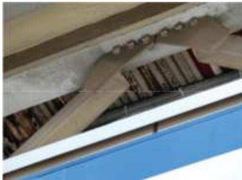
Plate 2.15 Out-of-plane deformation of gusset plate (Midorikawa et al, 2012)
