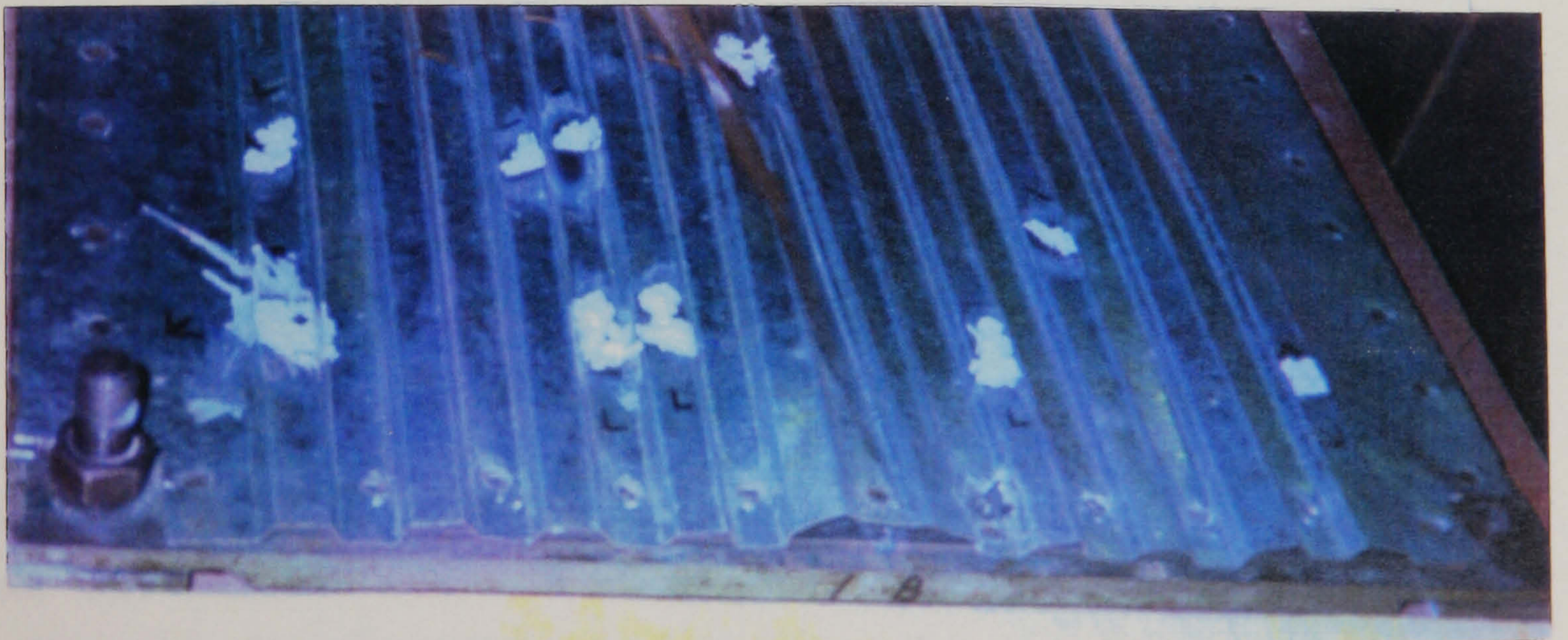
Photograph 5.4(b): Failure of the panel showing tearing of sheeting
