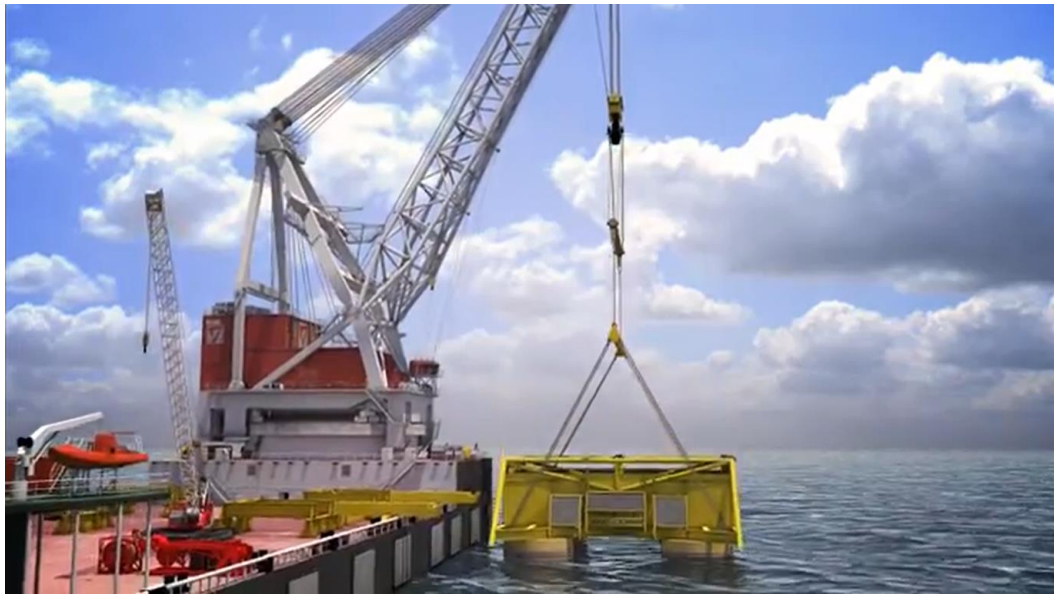
Figure 1.3-5 Subsea template lowering through splash zone (Braun, 2013)
