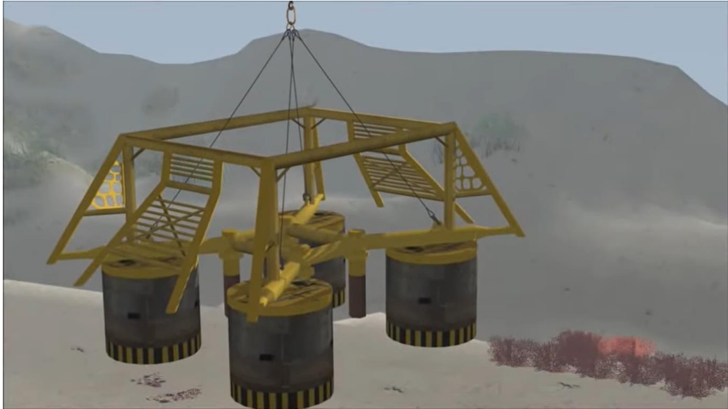
Figure 1.3-7 Subsea template lowered through water column to near-seabed (CM Labs, 2011)
