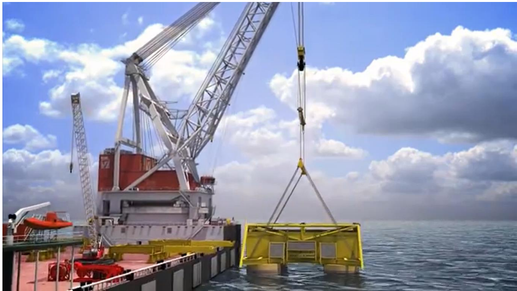
Figure 1.3-5 Subsea template lowering through splash zone (Braun, 2013)
