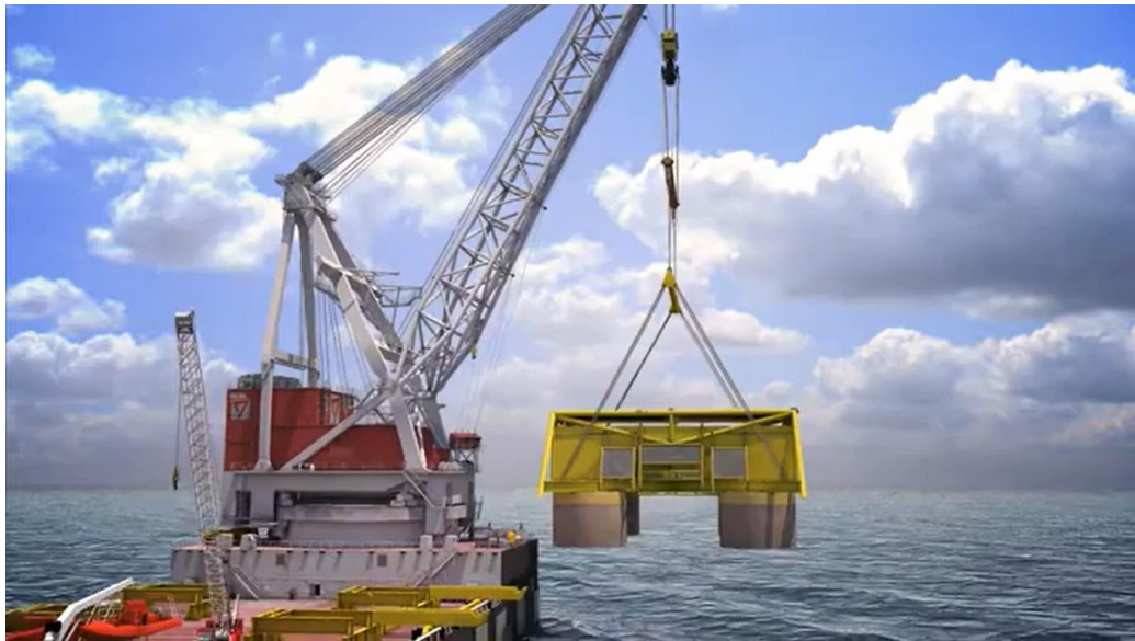
Figure 1.3-4 Subsea template over boarded and ready for lowering (Braun, 2013)
