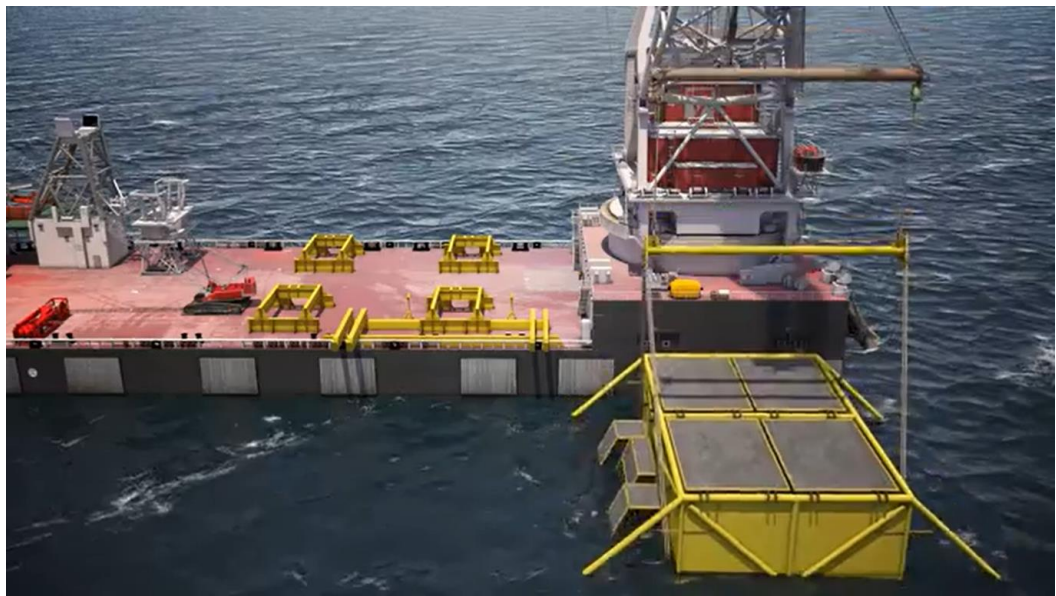
Figure 1.3-6 Subsea template lowering through splash zone (aerial view) (Braun, 2013)
