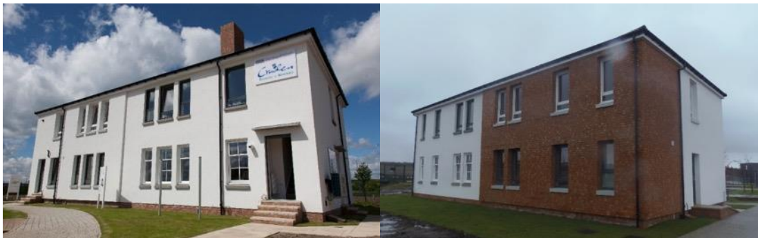
Figure 6.2: BRE Ravenscraig "Retrofit Building"
