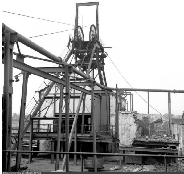
Figure 5.2: Headgear of one of the two original shafts at Cardowan Colliery, 1966 (Hume, 1966).
