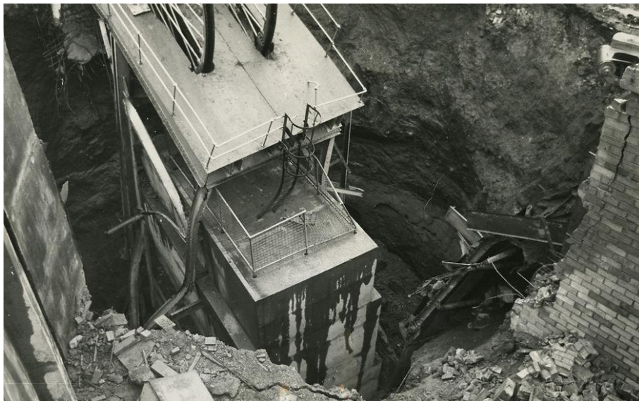
Figure 5.5: The Barony No.2 shaft its collapse in November 1962. Image from Perchard, 2020.
