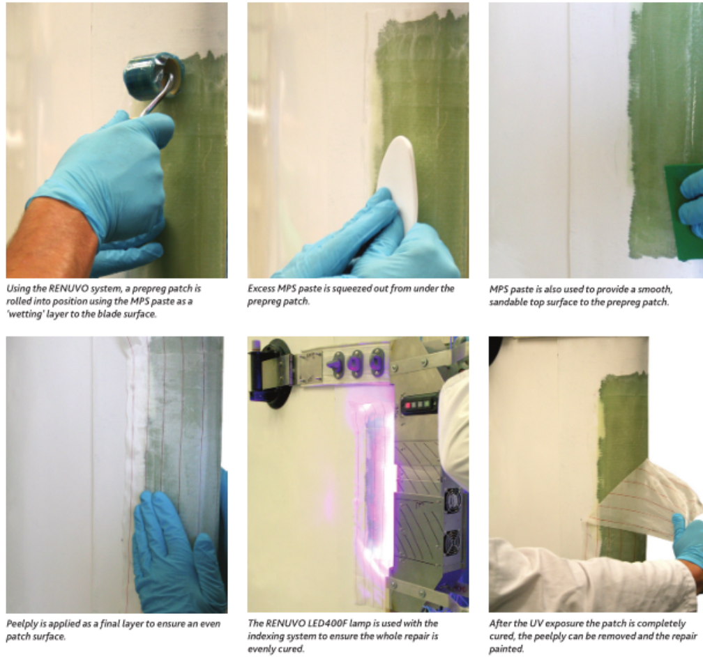
Figure 13: Stages of blade repair [10]
