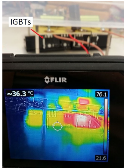
Figure 6.4: Thermal image of IGBTs in FB cell.
