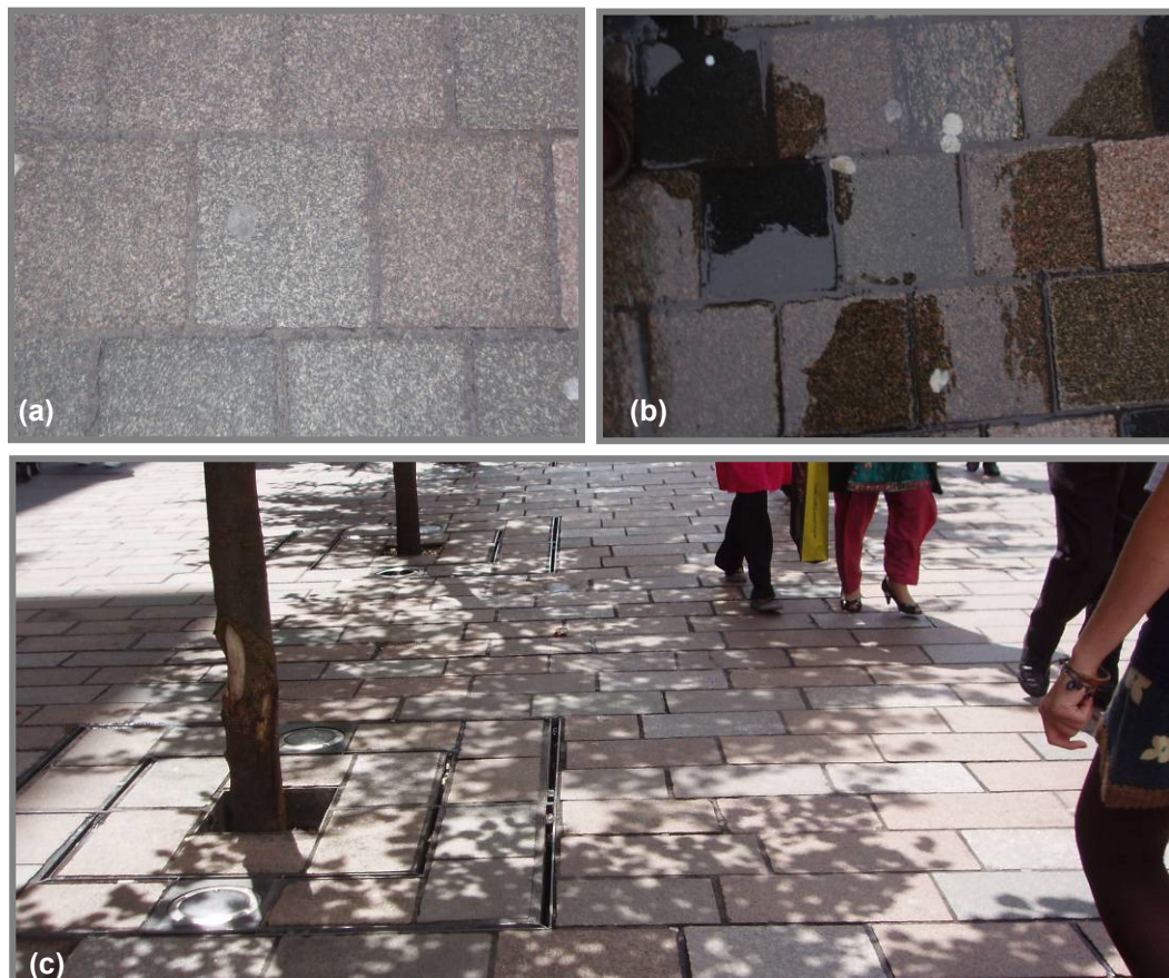
Figure 6.7: Pavement appearance under different weather conditions (a) Argyle St – dry, (b) Argyle St – wet and (c) Buchanan St – sunshine & shadow
