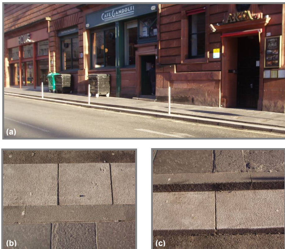
Figure 6.13: Double kerb along Albion St (a) Double kerb, (b) kerb as viewed from road and (c) kerb as viewed from pavement
