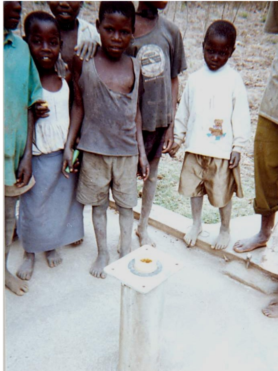
Ph.6.11 Vandalised "Kalika" borehole in Katundu 3 (Nov. 2006)
