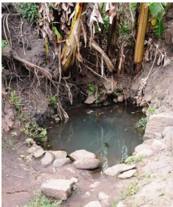
Ph. 2.1 Unprotected shallow well used by community in Mwitiwa Village, Thyolo (Aug.2007)
