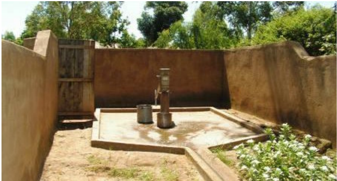
Ph.6.10 Katundu 3 "Portugal" borehole (Sept. 2006)
