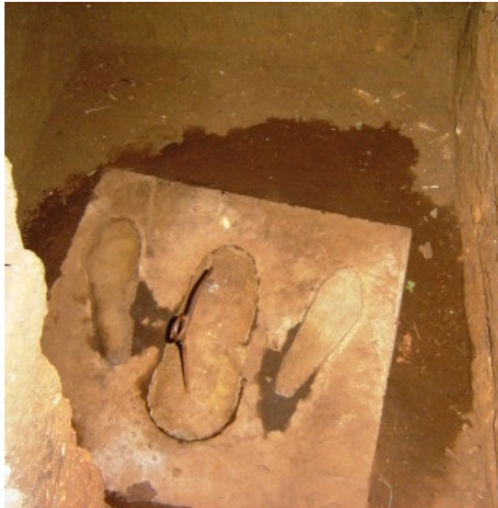
Ph. 2.8 A traditional pit latrine in Thyolo District, with a concrete slap (Sanplat) and cover (Nov. 2006)
