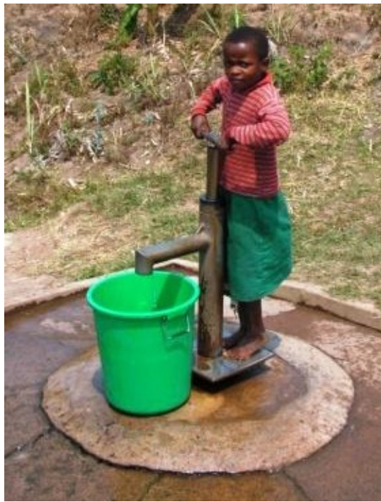
Ph. 2.4 Protected shallow well with Malda pump in Mwitiwa Village, Thyolo (Sept. 2006)
