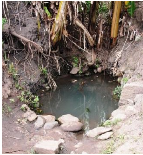
Ph.6.8 Unprotected shallow well, Mwitiwa (Aug. 2007)
