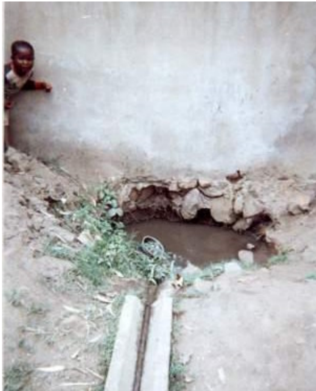
Ph.6.4 Soakaway of Katundu 3 "Portugal" borehole (Oct.2006)
