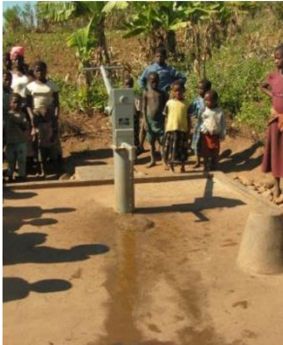
Ph. 2.3 Community borehole with Afridev pump in T/A Chimaliro, Thyolo District (May 2007)
