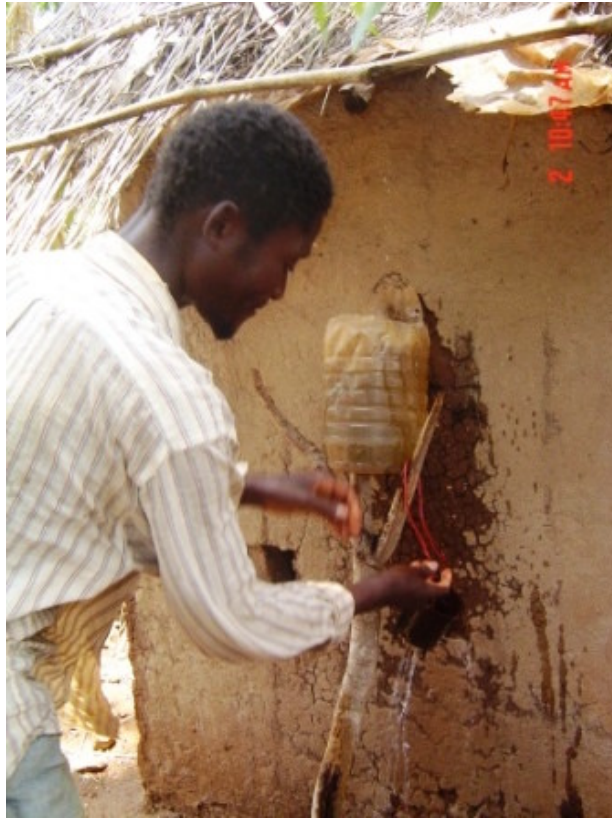
Ph.4.2 Simple handwashing facility using plastic container, a can and wire (Nov. 2005)
