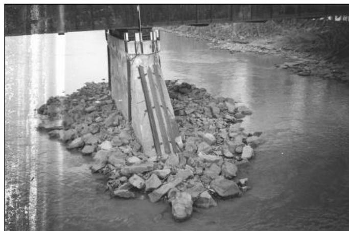
Figure 2-16: Sounding rods installed at a bridge pier [83].
