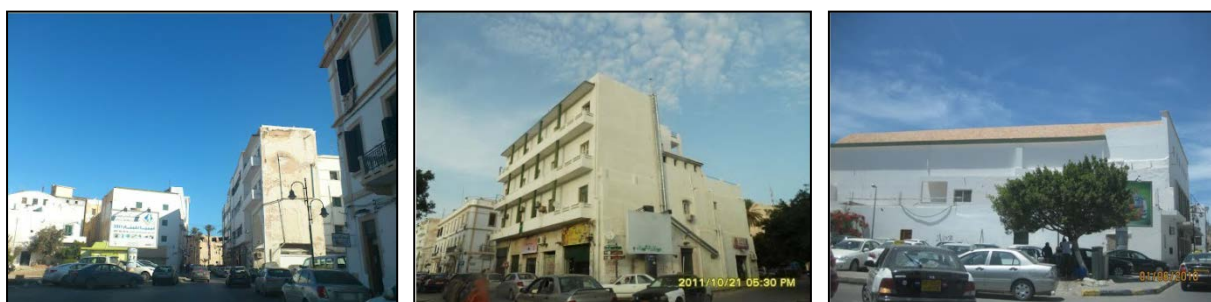
Figure 7.31: Bad street edges in the Italian Quarter
