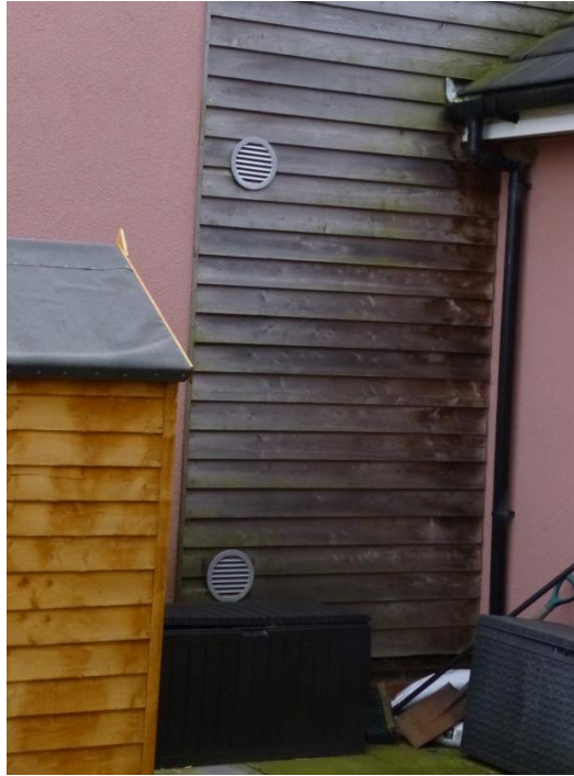
Figure 4.13: Intake and exhaust vents of the Dormont PH
