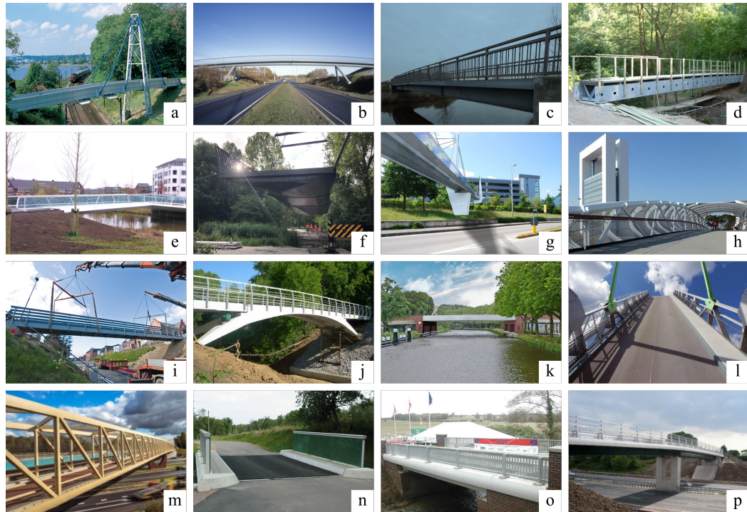
Figure 2.4: Applications of composite material in bridges. (a-j) pedestrian bridges. (k-p) road bridges. locations: Kolding, Denmark (a), Svendborg, Denmark (b), Esbjerg, Denmark (c), Grosseto, Italy (d), Harderwijk, Netherlands (e), Rotterdam, Netherlands (f), University of Salerno, Italy (g), Floriadeburg, Netherlands (h), Nørre Aaby, Denmark (i), Moscow, Russia (j), Delft, Netherlands (k), Karrebæksminde, Denmark (l), Utrecht, Netherlands (m), Klipphausen, Germany (n), Oxfordshire, UK (o), Lancashire, UK (p). Source of photographs: [17].
