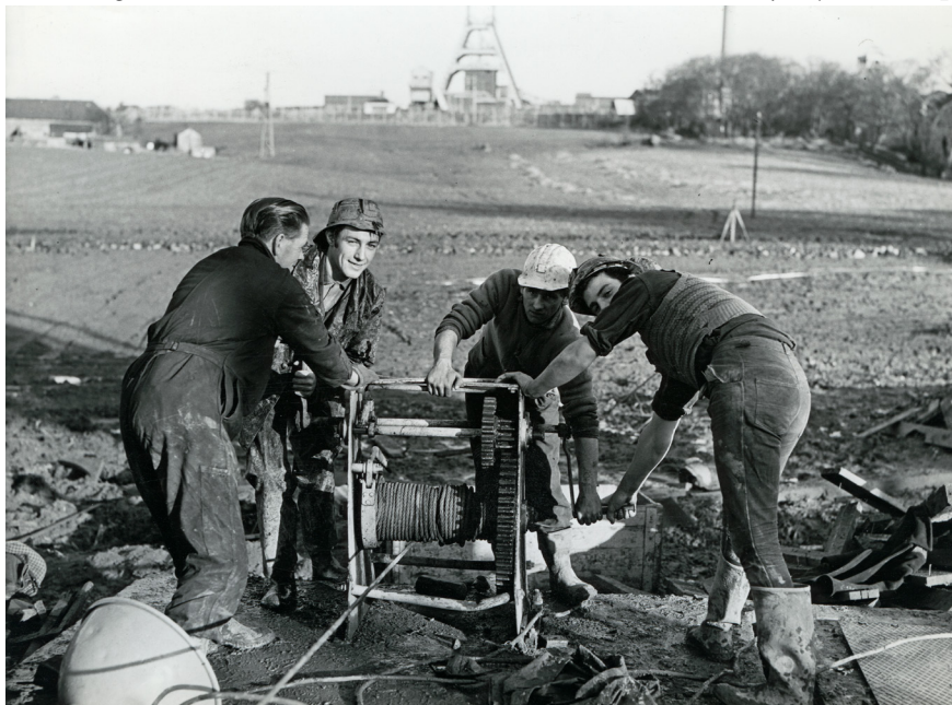
81: Men operating a hand winch at the Barony pit site (No. 4 sinking). The Barony A frame can be seen in the background. Courtesy of the National Mining Museum Scotland Trust
