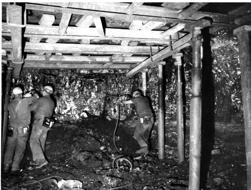
75: Working a relatively high seam at Pennyvenie, c. 1970. Note the safety helmets and the hydraulic props providing more robust roof support than pre-war. By kind permission of East Ayrshire Leisure Trust/East Ayrshire Council
