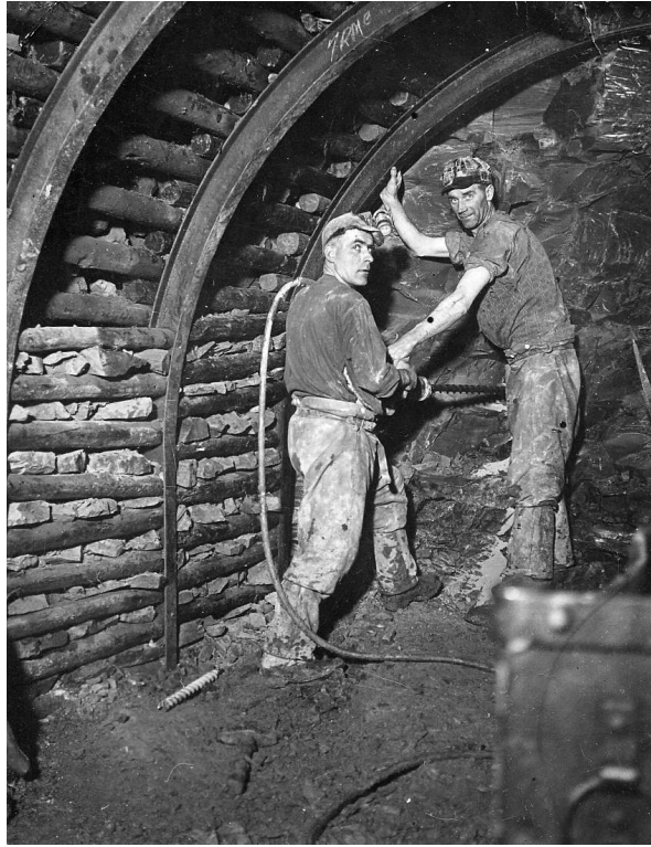
64: Miners working on cutting a new roadway through stone at the Chalmerston mine. Drilling for shot firing. By kind permission of East Ayrshire Leisure Trust/East Ayrshire Council
