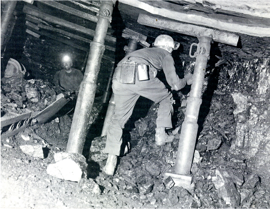
74: Coal getting underground using the pick at Pennyvenie. The steel props date this to the 1960s/70s.
