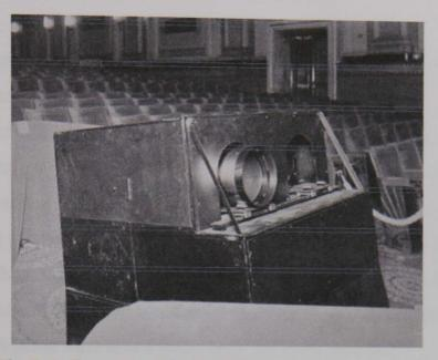
Fig. 7.10 Front view of the Baird Television projection machine showing the double projector as installed in the Marble Arch Pavilion, London Source: D. Brown
