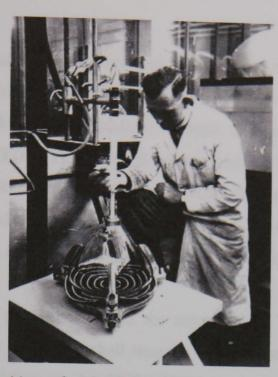
Fig. 7.20 Depositing a phosphorescent coating using the dusting technique at the Worsley Bridge Road Baird Television Limited factory Source: D. Brown
