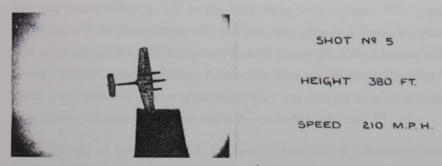
Fig. 7.14 *A trial recorded in AVIA 13/874 on the 14<sup>th</sup> of March 1939 of the photo-electric cell mounted in the nose of a Bristol Blenheim aircraft, serial L.1254. The aircraft being detected has the distinct outline of an Armstrong-Whitworth Whitley, although this type is not mentioned in the file.*
