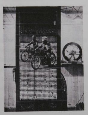
Fig. 7.2 The Screen used for the first cinema television demonstration (image is added) Source: Moseley, S. (1952). John Baird: The Romance and Tragedy of the Pioneer of Television. London: Odhams
