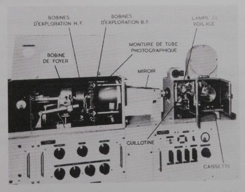
Fig 6.7 Ground receiver equipment supplied to French Government by Baird Television Ltd Source: R.M Herbert
