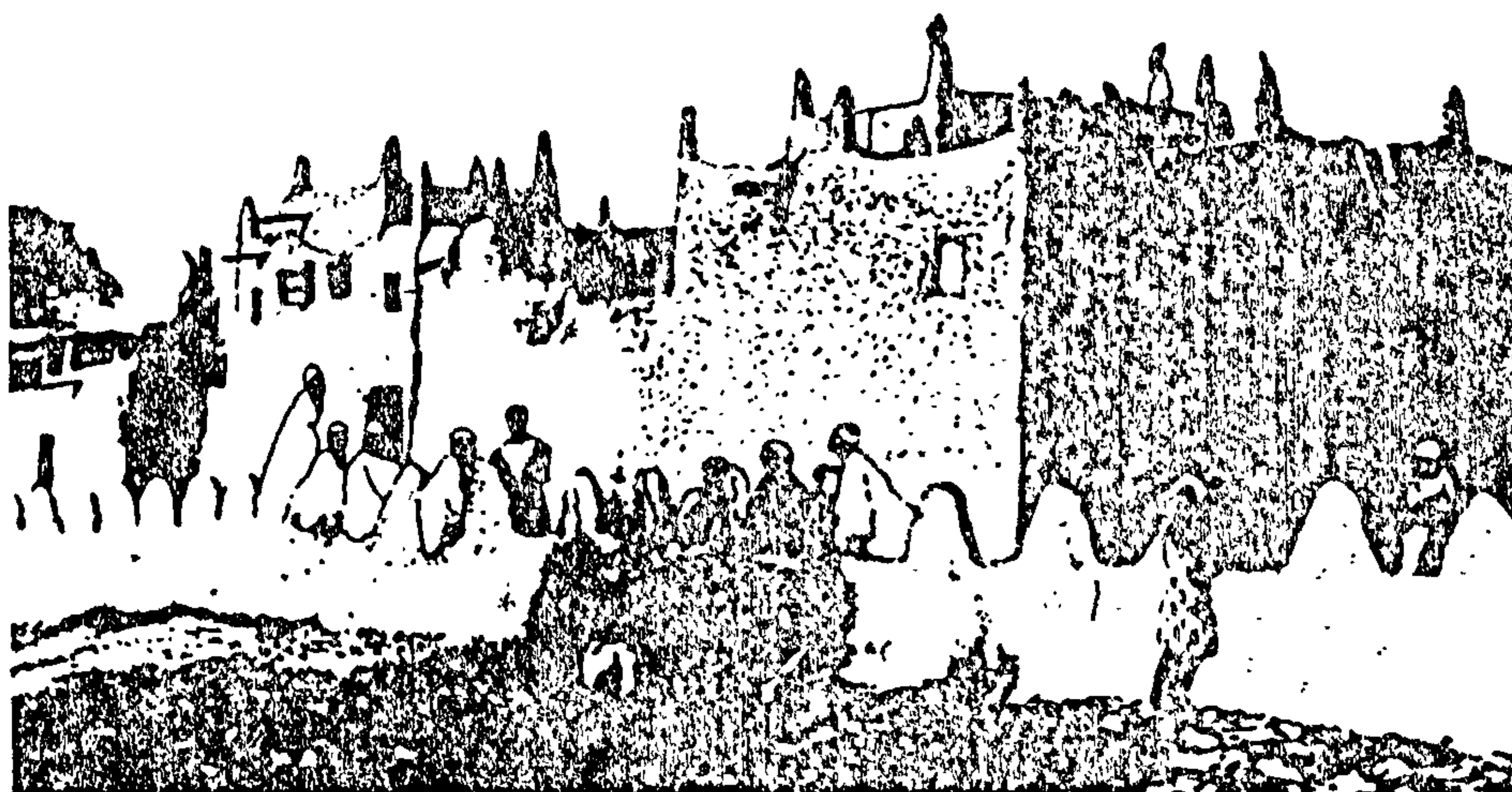
Fig. 3.10.B TRADITIONAL MUD HOUSES IN NIGERIA
