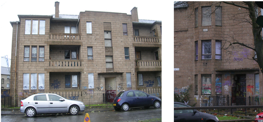
Figure 5.4: Example of local physical environmental conditions
