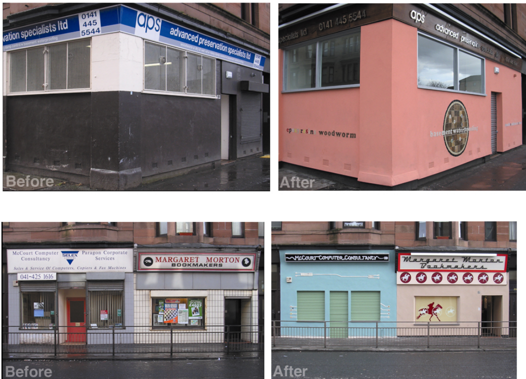
Figure 5.2: Example of improved shop fronts in local area
