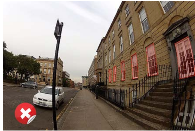
Figure 30 – Raised first-floor windows well above the street level and view of the pedestrian, which do not contribute to transparency quality (Location: Blythwood Sq.)
