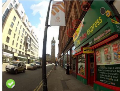
Figure 37 – 5 other lights integrated into the building facade. (Location: High St. 55°51'24.7"N 4°14'37.2"W)
