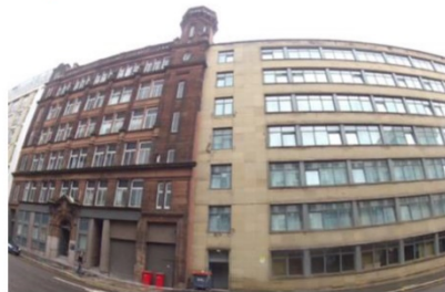
Figure 30 – Floors of the building on the right are approximately 3m high, so the total building height is approximately 21m. The building on the left has a higher
