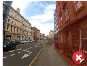
Figure 40 – The building is inactive with no visible activity at street level. (Location: Bath St. 55°51'50.4"N 4°15'27.6"W)
