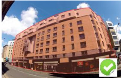
Figure 14 – A building with nonrectangular shapes (Location: High St. 55°51'24.7"N 4°14'37.2"W)
