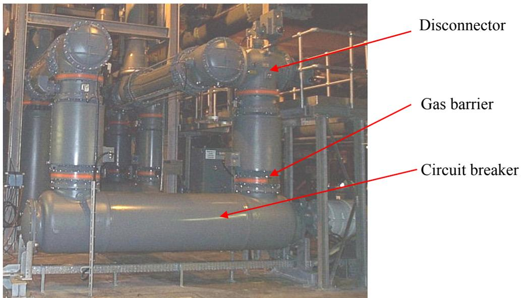
Figure 2.11: Photograph showing an SF<sub>6</sub> gas insulated circuit breaker
