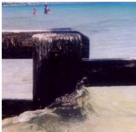
Figure 2.3 Illustration of the wave run-up resulting from an incident wave impinging on a vertical surface piercing column (Morris-Tomas et al., 2004)
