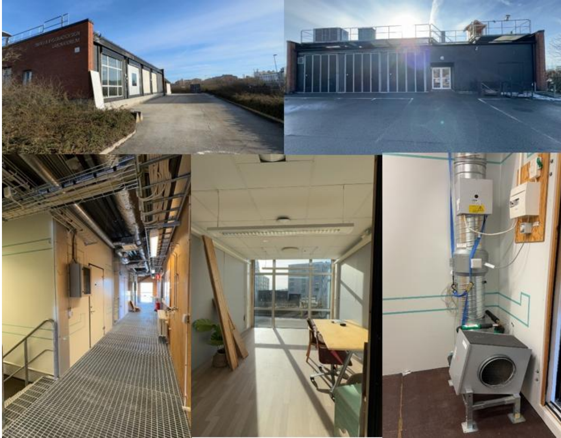
Figure 5.1: North and south facades of the EBD Laboratory (top left: north facade; top right: south facade), circulation area (bottom right), one of the lighting cells (bottom middle), and one of the thermal cells (bottom left)
