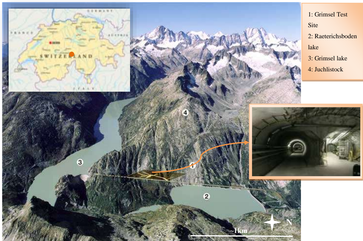
Figure 2: Panoramic picture of the general area where the GTS sits. Insets show the location of the GTS in Switzerland (in an orange dot) and a photograph from inside the main tunnel. Figure adapted from http://www.grimsel.com/gts-phase-vi/lasmo/lasmo-project-perimeter-gts-layout
