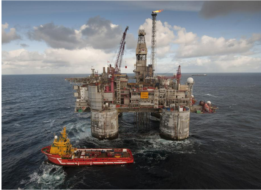
Figure 1.1: Production TLP on Statoil's Heidrun field, Norwegian Sea. Courtesy of www.offshoreenergytoday.com .
