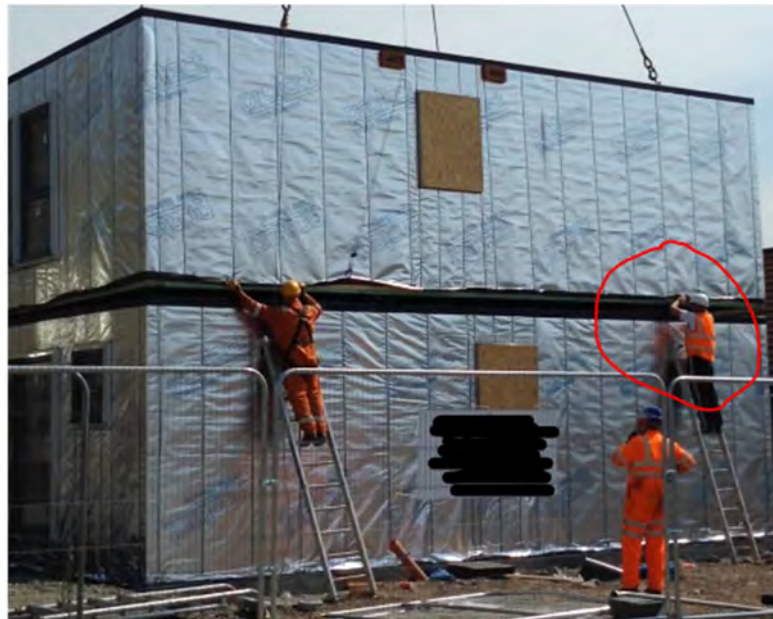
Figure 92. High-risk activity near-miss installation scenario instance marked in red.
