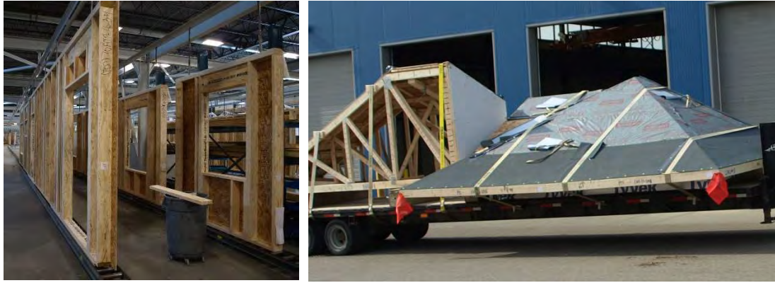
Figure 77. Laminated Strand Lumber panels and a modular roof observed in Canada.
