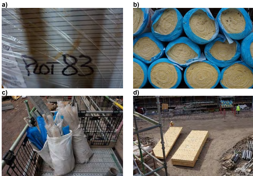
Figure 7B15. CTP case study materials waste and storage observations: a) plasterboard, b) insulation, c) packaging, d) just-in-time panels delivery.
