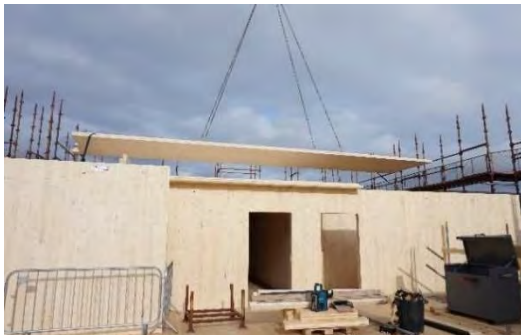
Figure 7B4. Floor panel CLT installation.
