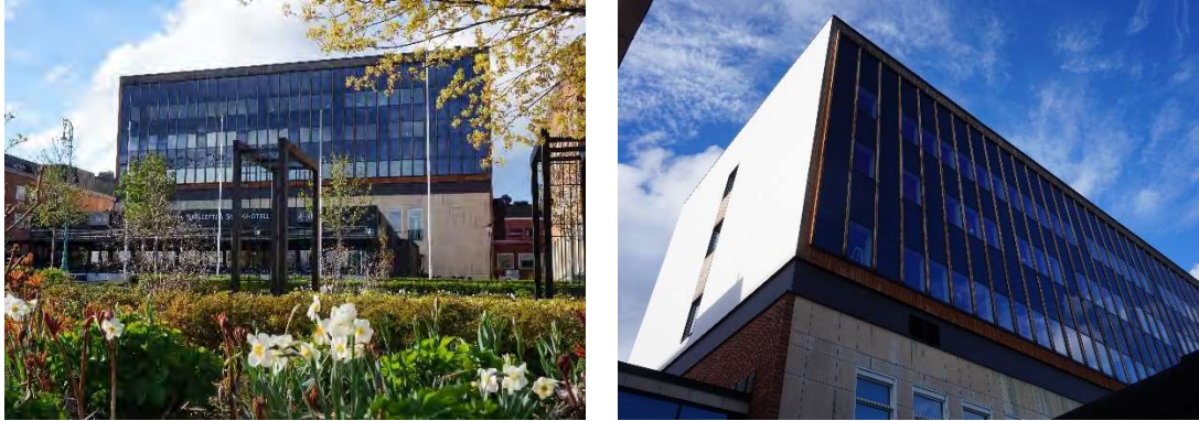
Figure 83. Hotel with lightweight CLT extension of four storeys. Author's own images. June 2017.
