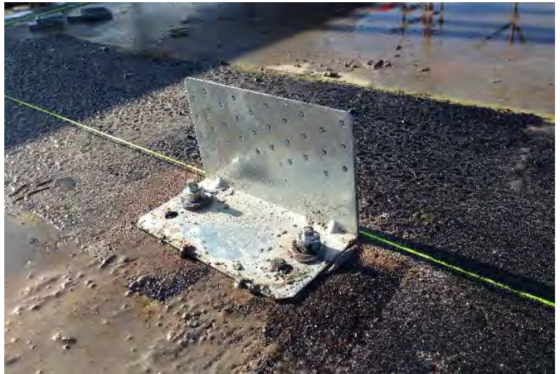
Figure 7B2. CLT ground floor brackets.
