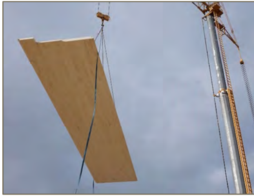
Cross-laminated timber panel
