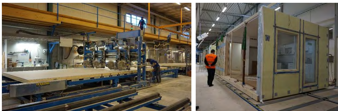
Figure 81. Volumetric timber manufacturing process in Sweden: panelised and modules. Author's own images. June 2017.
