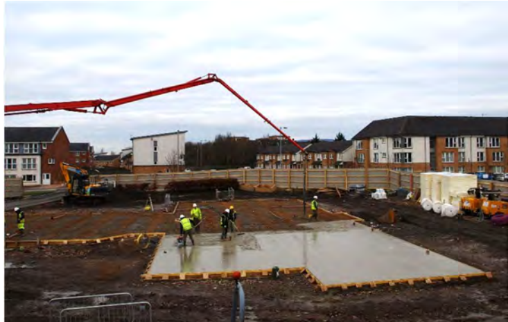
Figure 7B1. CLT floor slab.
