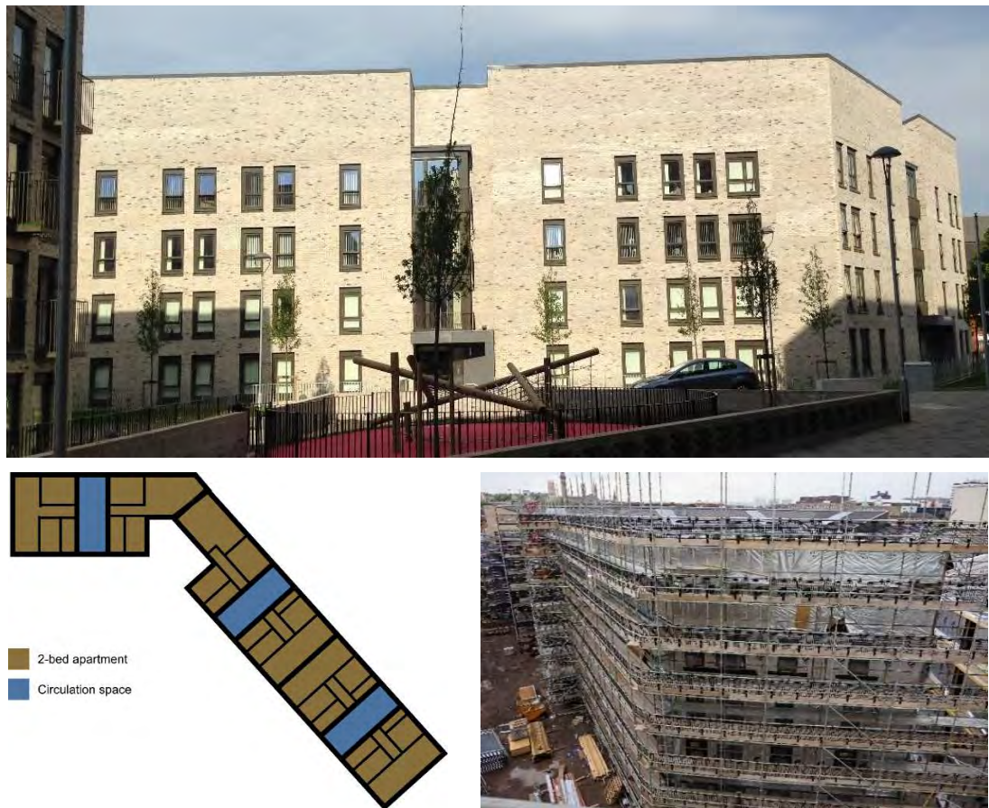
Figure 95. CTP project: overview, typical layout and during construction.
