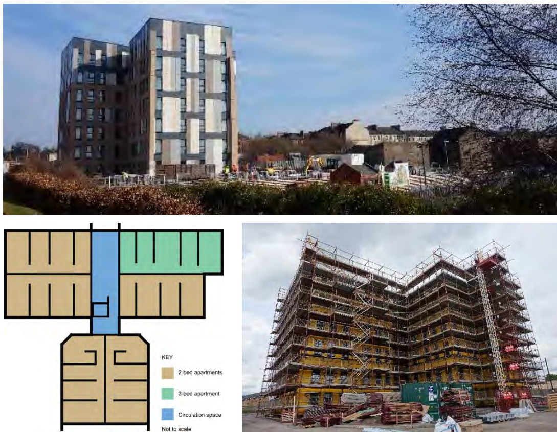
Figure 94. CLT project: overview, typical layout and during construction.
