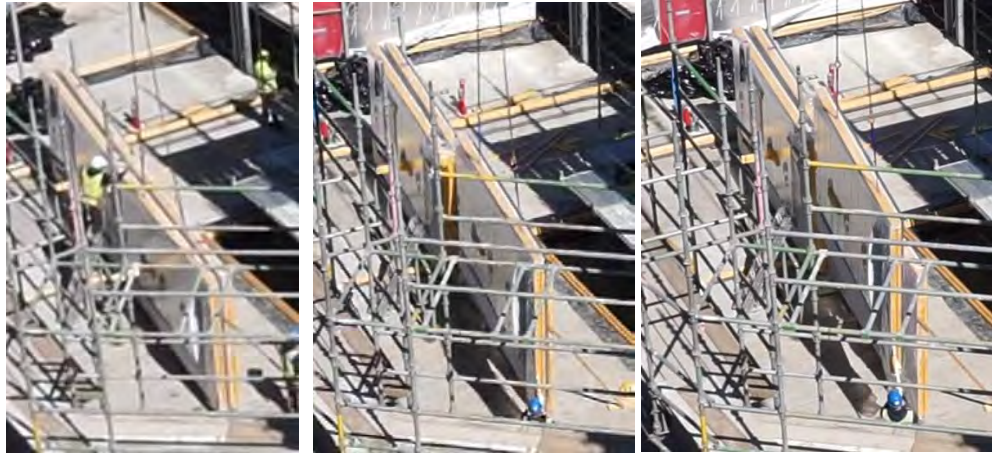
Figure 7B17. Two-in-one transporting and lifting system used in CTP project.
