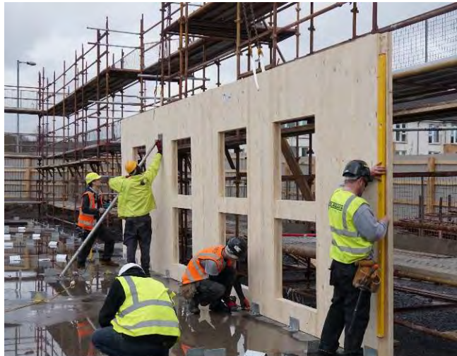
Figure 7B3. CLT wall panels.
