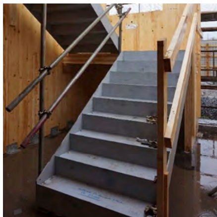
Figure 7B10. Staircase at CLT case study. 17/03/2017 DSC00616.
