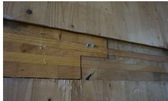
Figure 7B5. Floor panel CLT connection.
