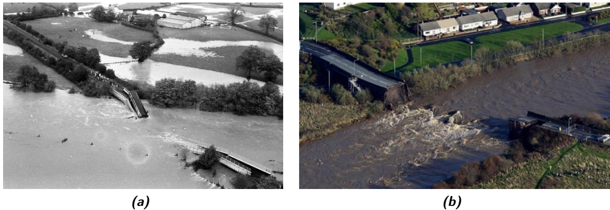
Figure 2.8: (a) Glanrhyd railway bridge disaster in 1987 in Wales (Huw Evans Agency, 1987) and (b) an aerial view of the destroyed Northside bridge in Workington (Cumbria) in 2009 (Byrne, 2009)
