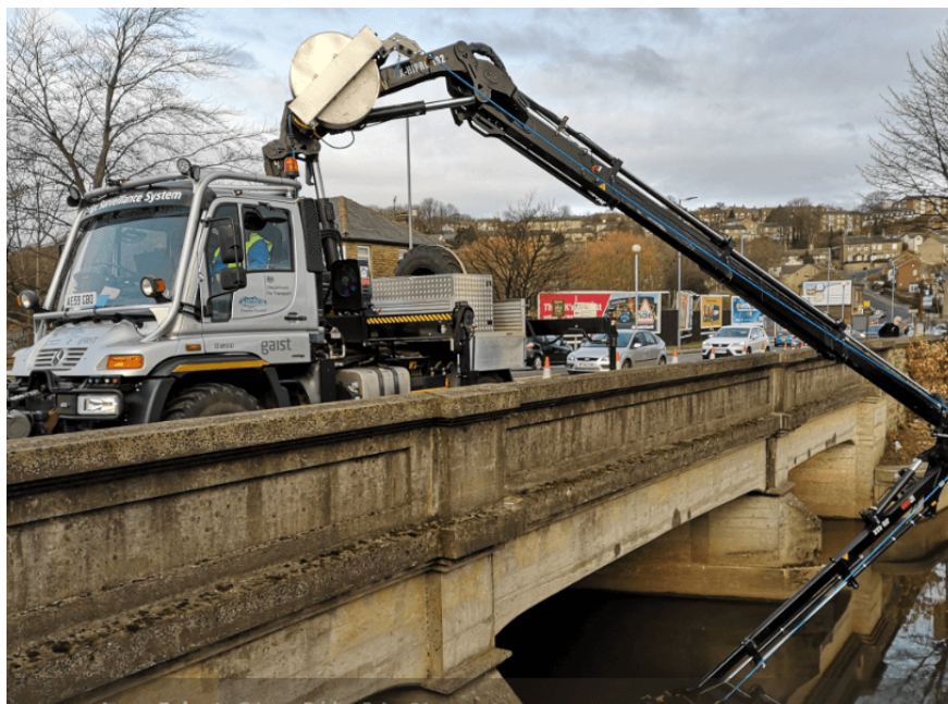
Figure 2.13: Bridgecat technology for bridge inspection (PCSG, 2019)
