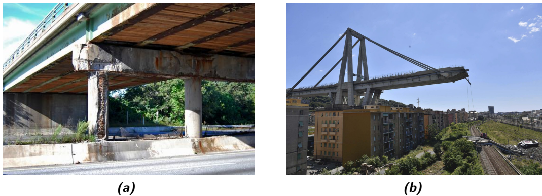
Figure 2.1: (a) Long-term deteriorations make the steel reinforcement visible in piers and beams ( The Boston Globe, 2009 ) and (b) the collapsed Morandi bridge in Genova in the 2018 ( The Guardian, 2019a )
