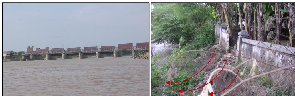
Figure 2.9: (a) Babat barrage and (b) rapid drawdown failure at Plangwot village
