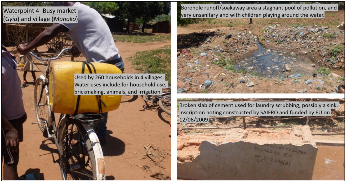
Figure 5.52: Waterpoint with evidence of polluted runoff pool, and degraded infrastructure.
