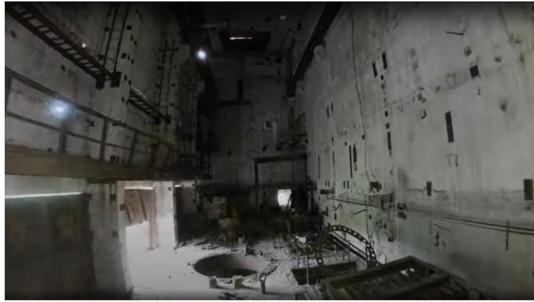
Figure 1-4: Example of reconnaissance to determine the state of an enclosed structure. Here exploration and monitoring of an unused holding pool building is conducted within the Chernobyl nuclear power plant [46].
