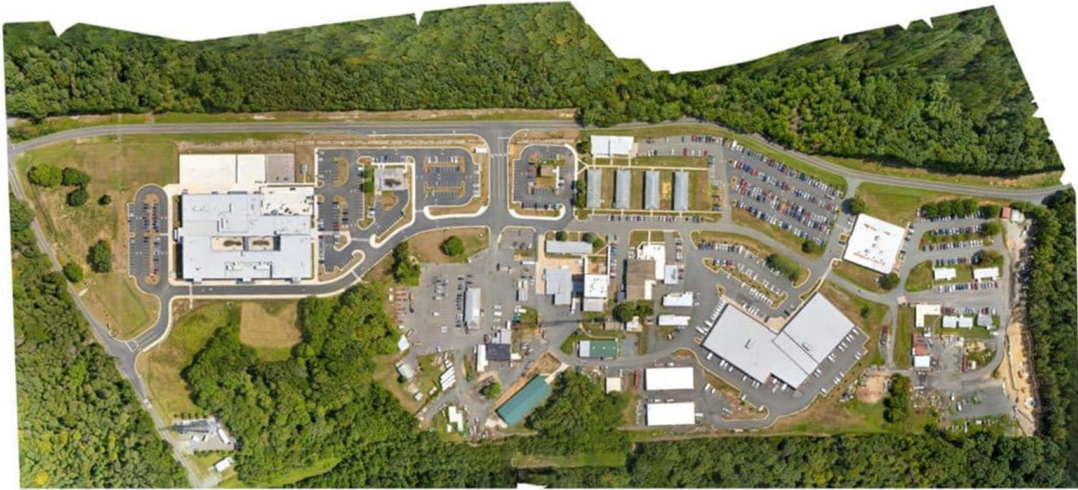
Figure 2-2: An example of an aerially captured orthoimage of a light industrial facility [131]. Minor distortions are visible at the image extremes owing to the repeating texture and incomplete geometry capture of the trees on the property boundary.
