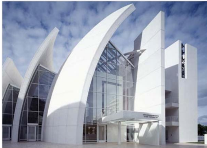
Figure 1.2: Jubilee Church in Rome: (Source: quartiermagazin.com/quartier08/der-weise-riese ).
