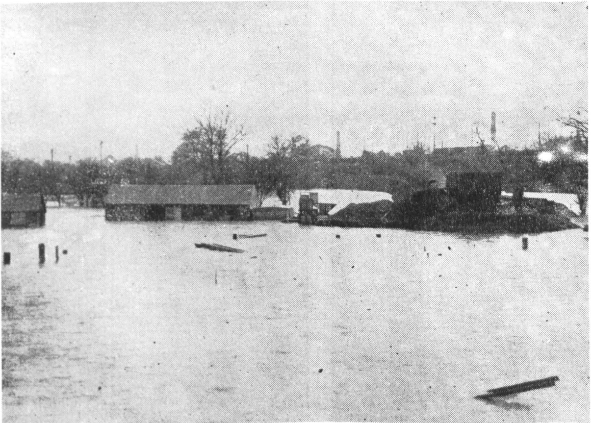
Plate II. Carlisle: The new electricity works under construction at Willow Holme - flooded in January 1925.
