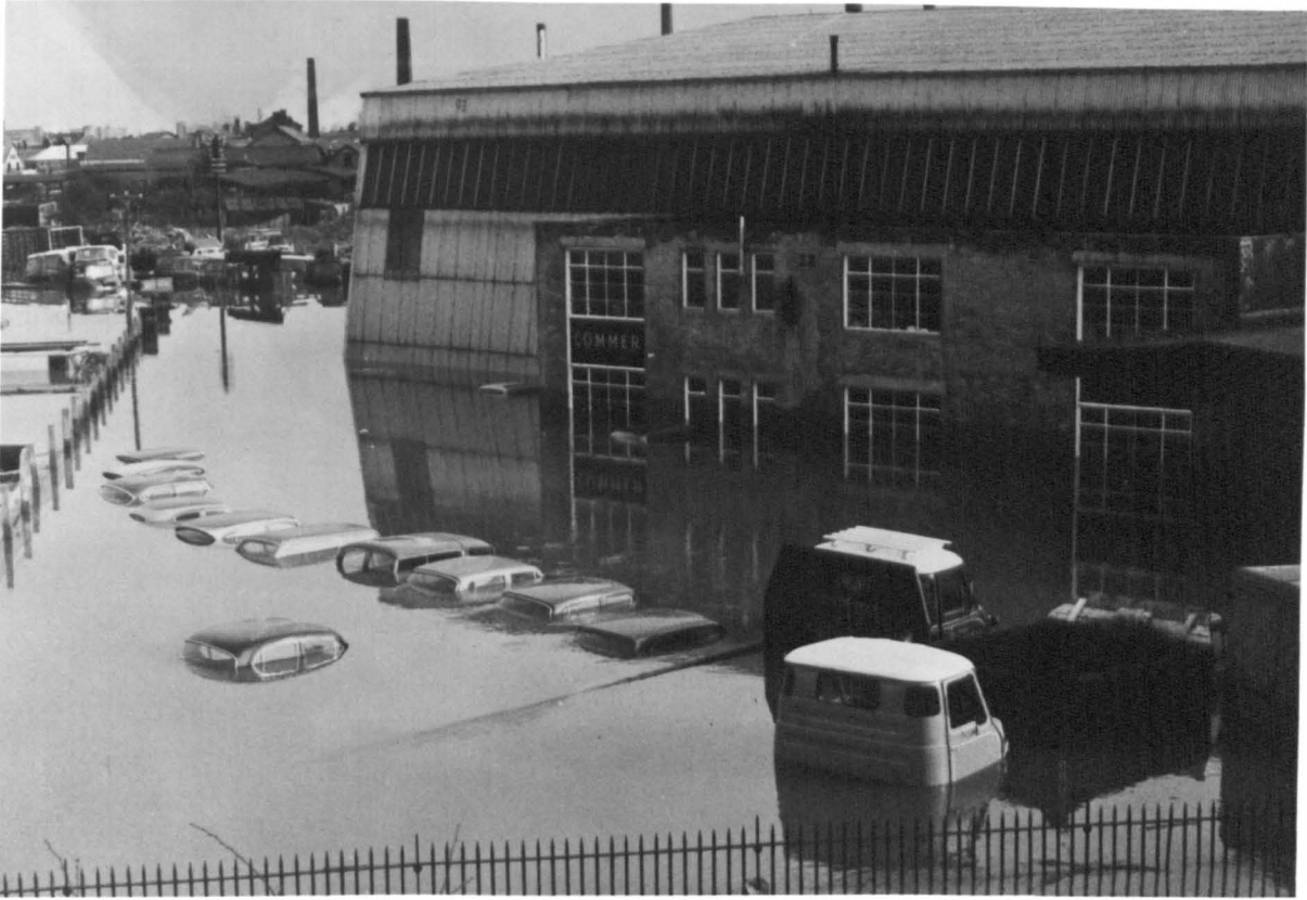
Plates 25 and 26. Carlisle: The flood damage at McKenzie's Motors (Willow Holme Industrial Estate) several hours after the peak discharge.
