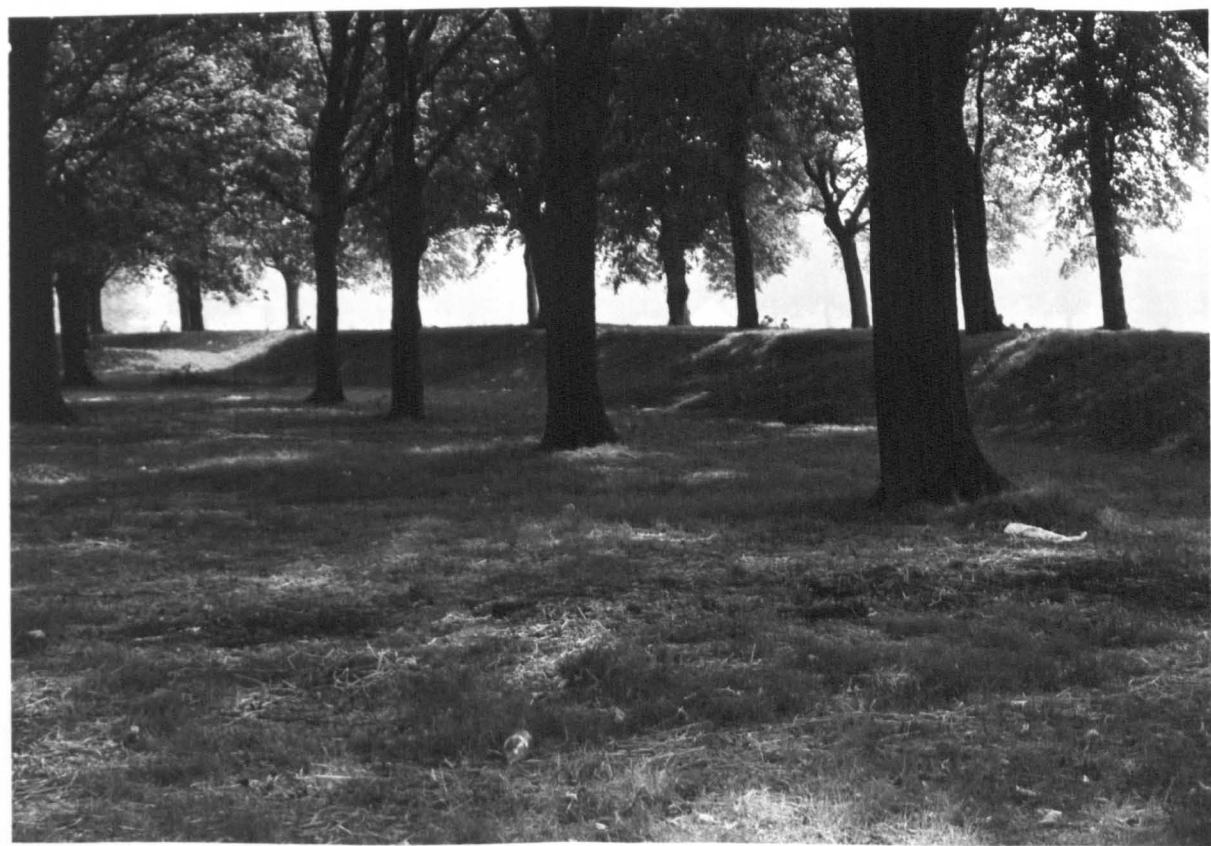
Plate 16. Carlisle: Part of the flood embankment scheme on the Saucerries.
