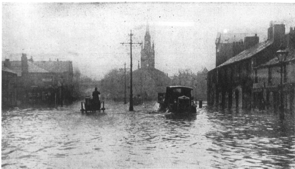
Plate 12. Carlisle: Flooding of Church Street in Caldewgate in January 1925.
