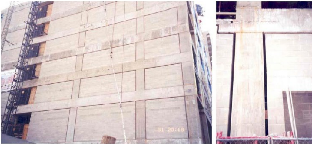
Figure 2.16. Introduction of gaps in the infilled frame system (Aliaari and Memari 2005).
