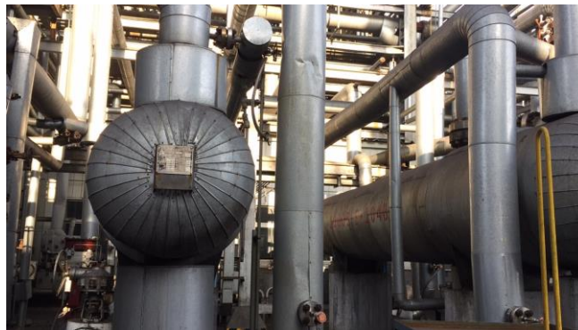
Fig. 1.1. Heat exchanger under high pressure and elevated temperature conditions in energy industry
