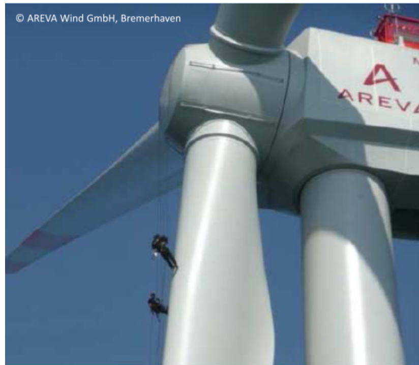
Figure 2.37: Technicians inspecting a turbine blade via rope access [27].
